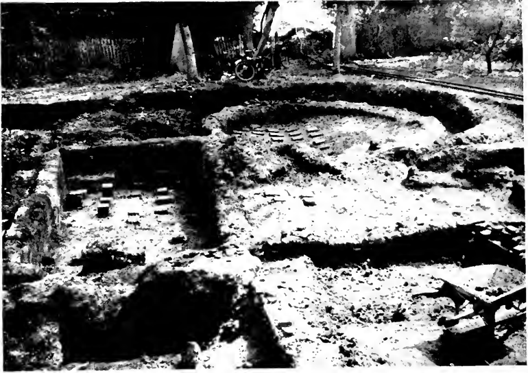
BATH HOUSE, LOOKING S.E.
