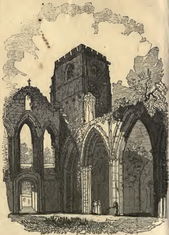
Interior of the Nave, LANDAFF CATHEDRAL.
