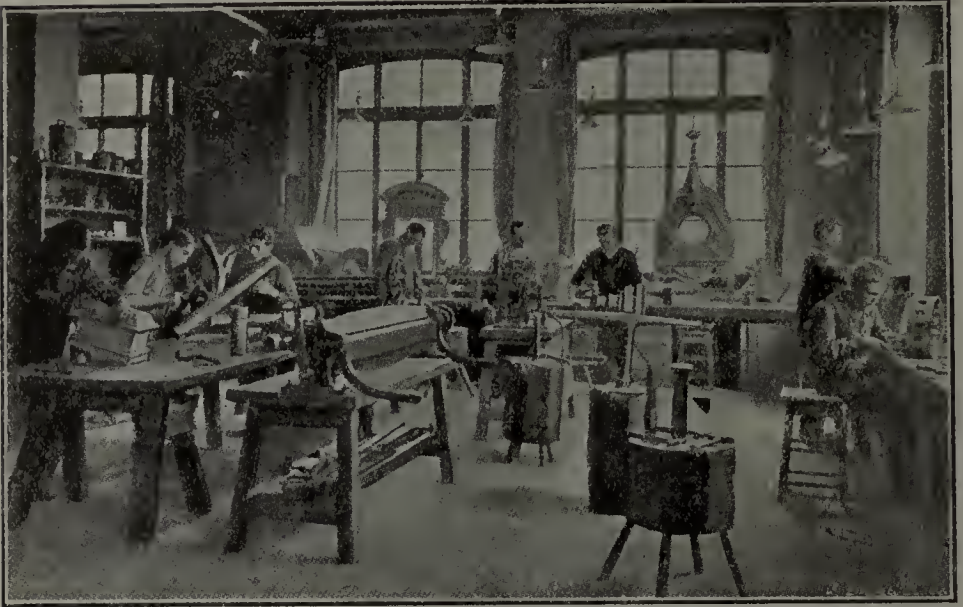
TINSMITHS' AND PLUMBERS' WORKSHOP: INDUSTRIAL ART SCHOOL AT GENEVA.
