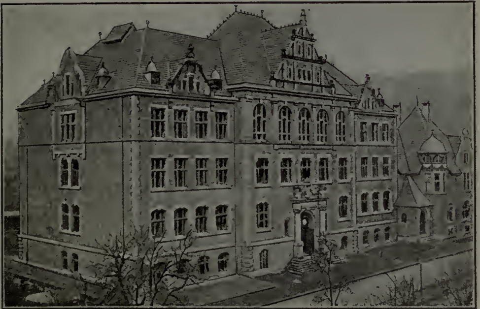
THE ROYAL BUILDING TRADES SCHOOL; BARMEN-ELBERFELD.
