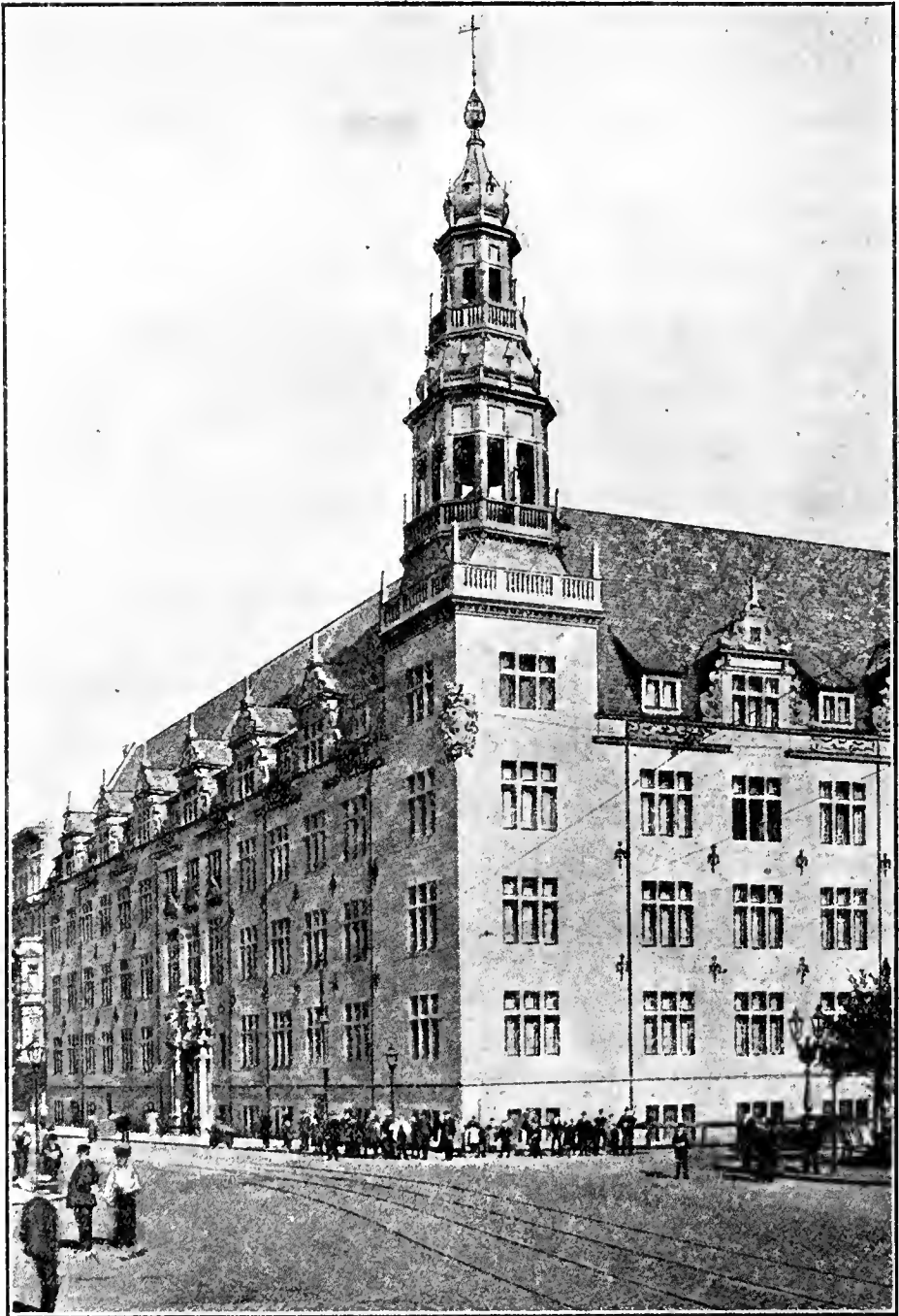
GENERAL VIEW OF A HANDWORKERS' SCHOOL : BERLIN.
