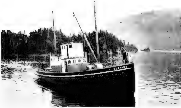
SELDOVIA SALMON CO.'S TENDER GLOVINA. This Is the Most Recently Constructed of the Cannery Tenders.
