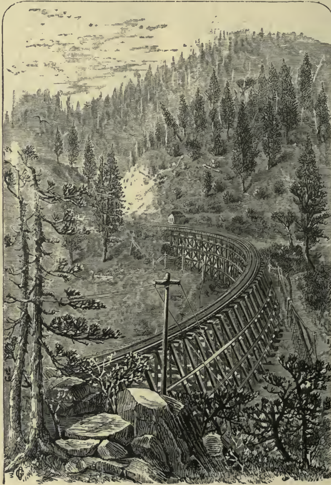
SECRET TOWN, TRESTLE WORK.
