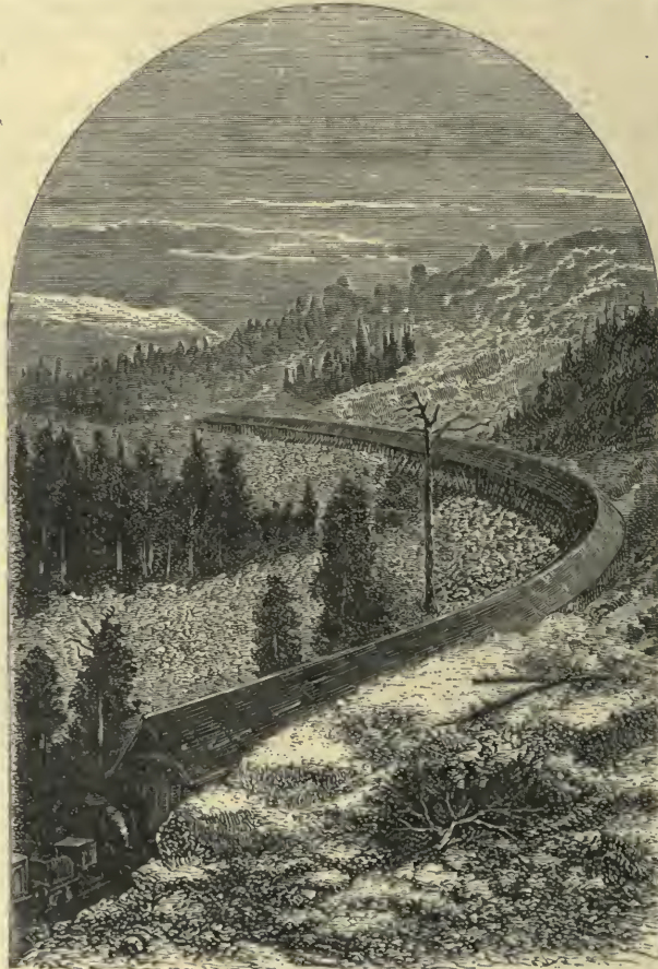
SNOW SHEDS ACROSS THE SIERRAS.
