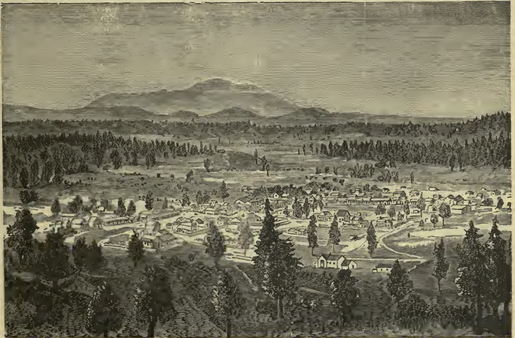
VIEW OF PRESCOTT, CAPITAL OF ARIZONA.
