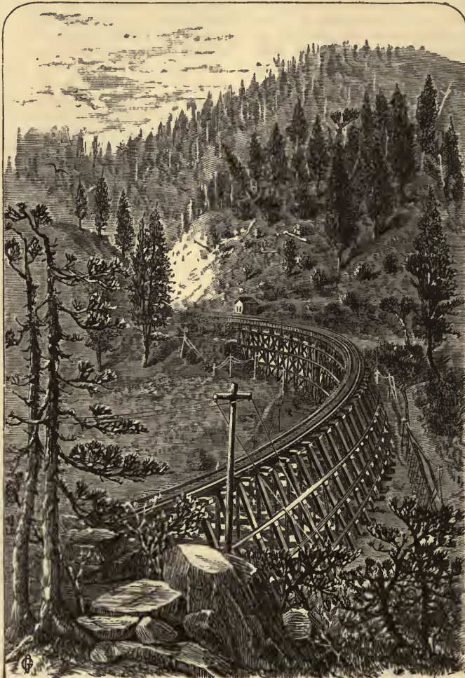
SECRET TOWN, TRESTLE-WORK.
