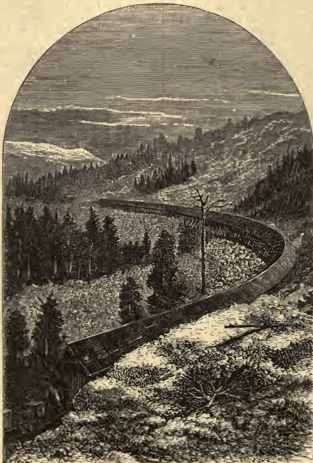
SNOW SHEDS ACROSS THE SIERRAS.
