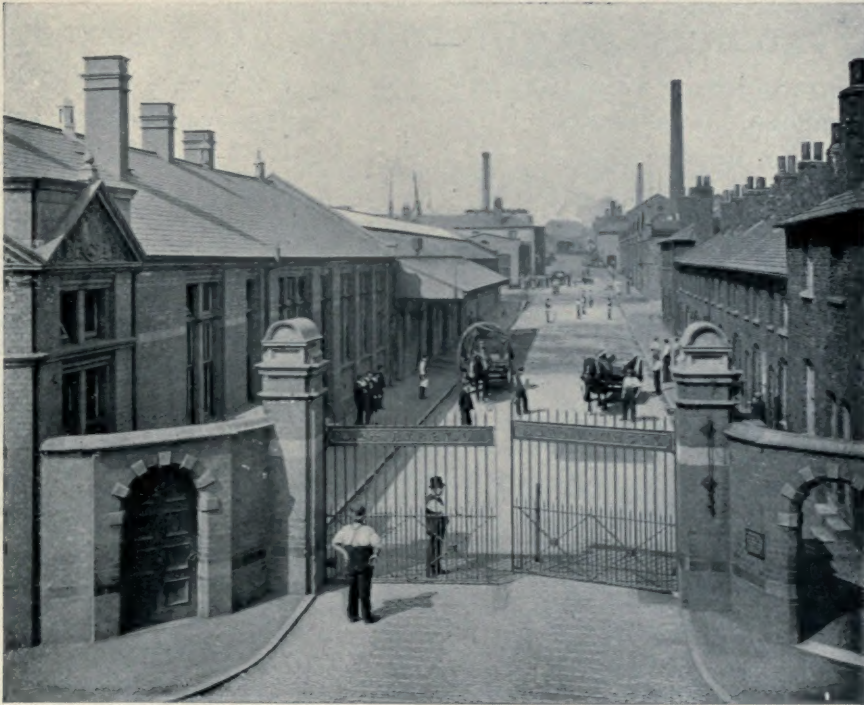
Entrance to Avery's Main Works, Soho Foundry, Birmingham.
