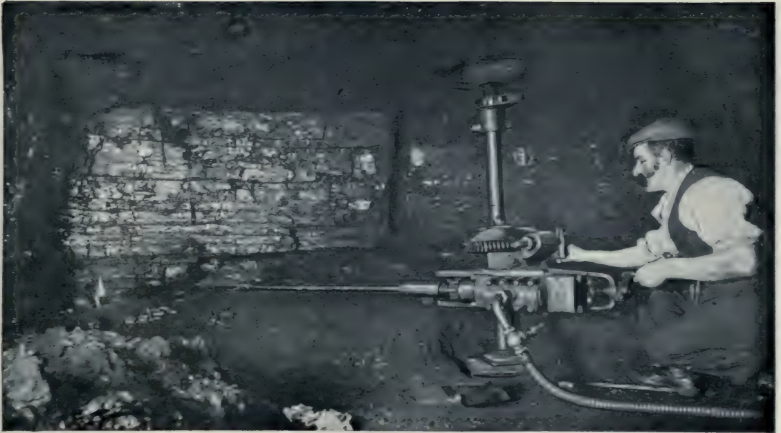
ILLUSTRATION SHOWING SHEAR AND UNDERCUT FINISHED.
