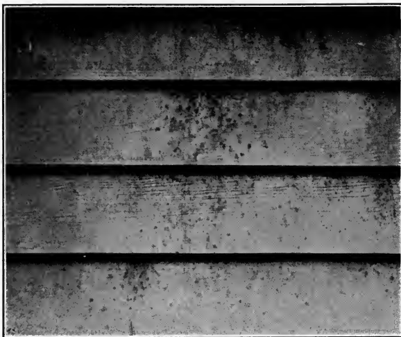
FIG. 120. Section of Dwelling Showing Growth of "Mildew."
