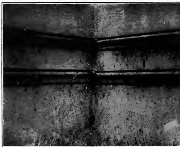
FIG. 121. Appearance of Painted Surface Marred by Fungous Growth.
