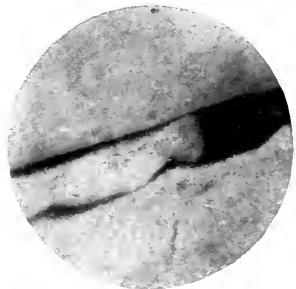
18. Effect of Cracking on Hard Pine, Causing Splitting of Painting Coating
