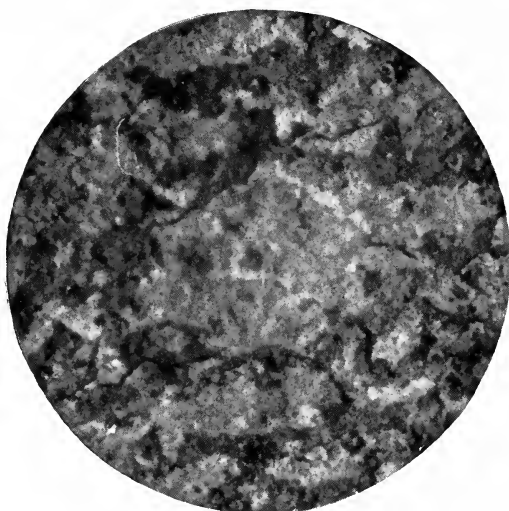
Formula No. 36, Pittsburg Basic Carbonate — White Lead Panels on Fence
