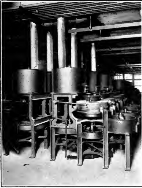
Battery of Paint Mixers and Grinders of Modern Underdriven Type
