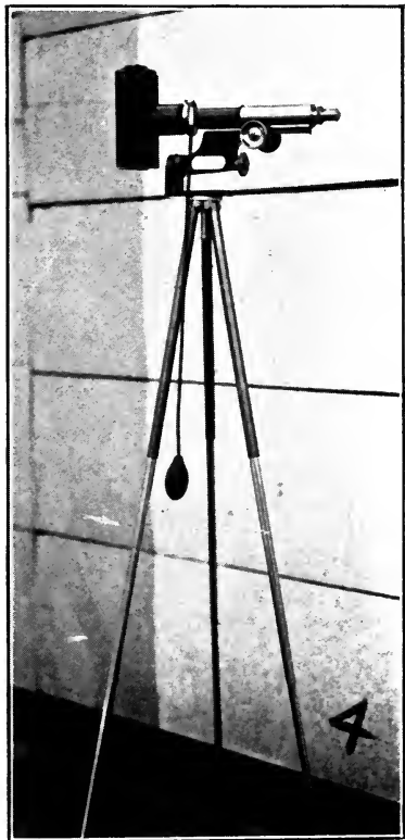
Gardner photomicroscope in position against painted surface
