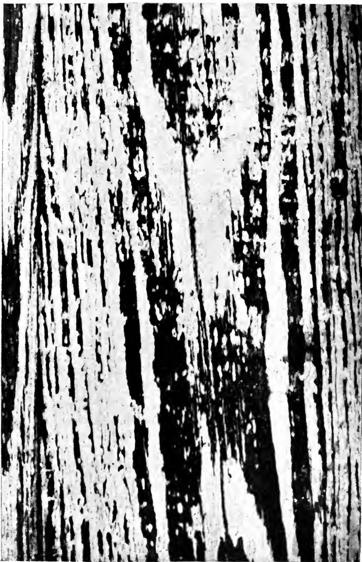
SCALING. — Type of Decay Exhibited by Improperly Made Paint (magnified view)
