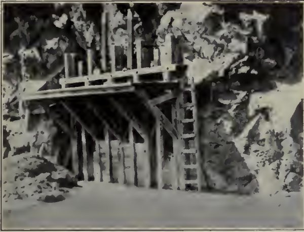
Headgates of Canal
