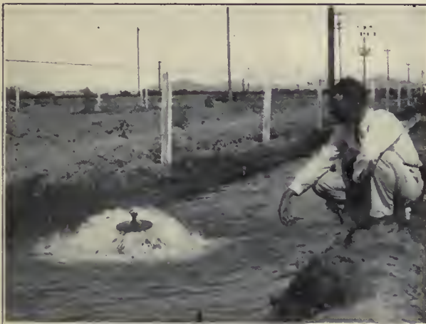
Hydrant With Cap On
