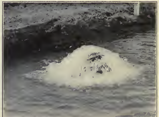
Hydrant With Cap Removed
