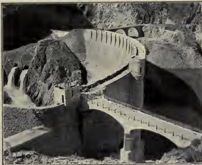
Roosevelt Dam, Solid Granite, Built on Granite, Locked Into Granite. Furnishes Electrical Power for Palmborg Colony
