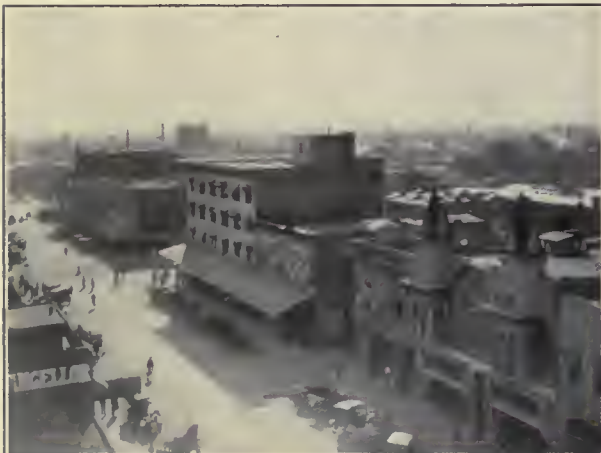
Part of Business Section of Phoenix
