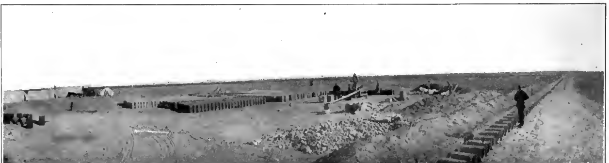
This Is One of the Cement Pipe Plants, Making the Concrete Conduits on the Ground, for Carrying the Irrigating Water to All Parts of the Palmborg Colony
