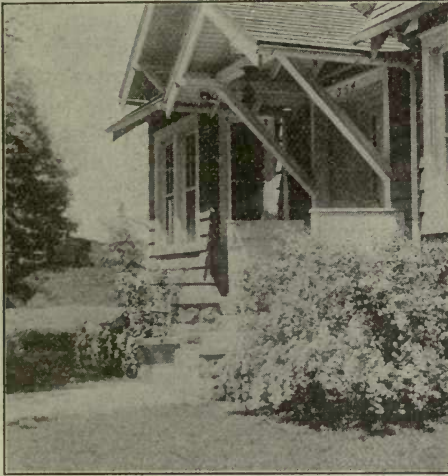
Shrubs planted in the corners of the entrance porch generally prove effective.
