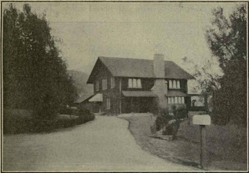
FIG. 32.—A satisfying result with a slightly curved roadway, a deviation of not more than its own width.
