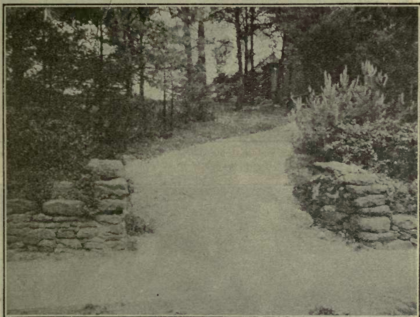
FIG. 24.—A well-designed entrance. The appearance of the stone wall has been improved by recessing the cement joints.
