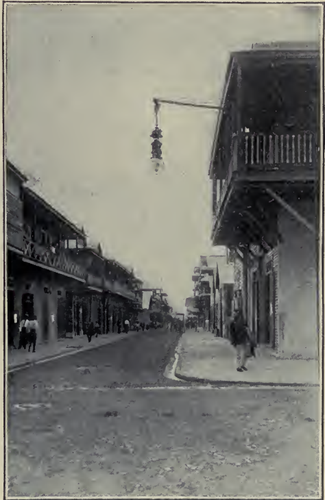
STREET IN COLON—PAVED AND CLEANED.
