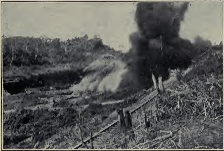
EXPLOSION IN PROGRESS, MATACHIN.—19 HOLES, 11,200 POUNDS DYNAMITE, 17,980 CUBIC YARDS DISPLACED, JANUARY 10, 1908.
