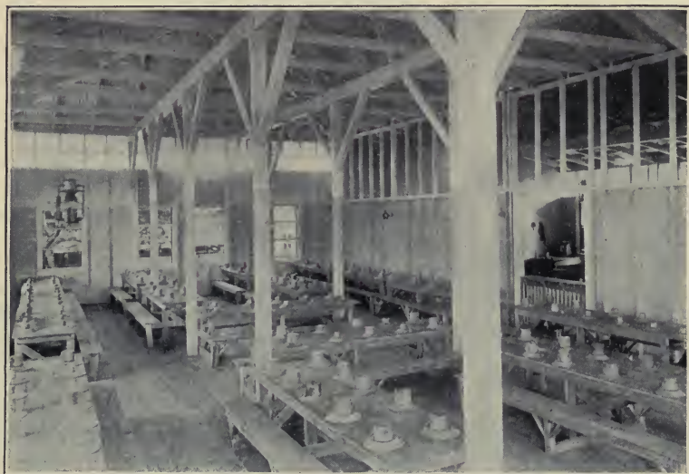
INTERIOR OF A MESS HALL FOR EUROPEAN LABORERS.
