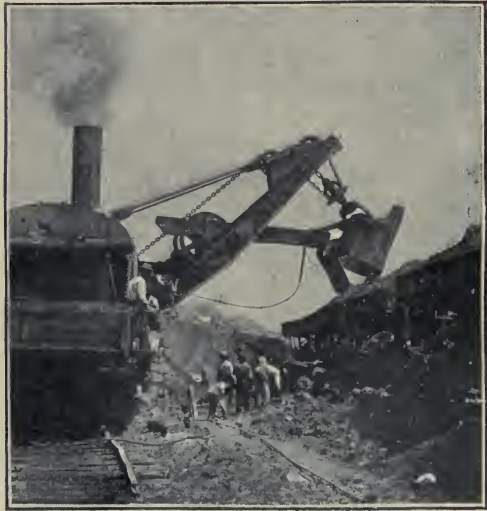
STEAM SHOVEL—SHOWING ARM AND DIPPER.
