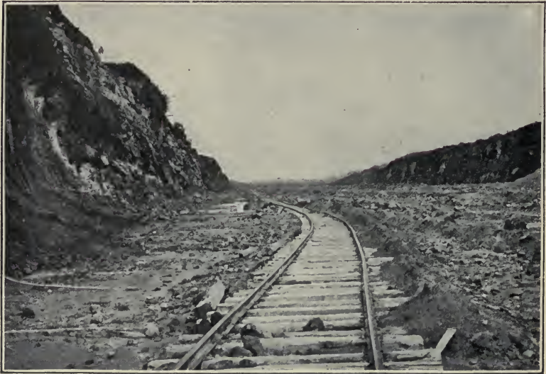
EXCAVATION FOR GATUN LOCKS COMPLETED.
