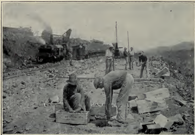
LOADING DRILL HOLES WITH DYNAMITE.
