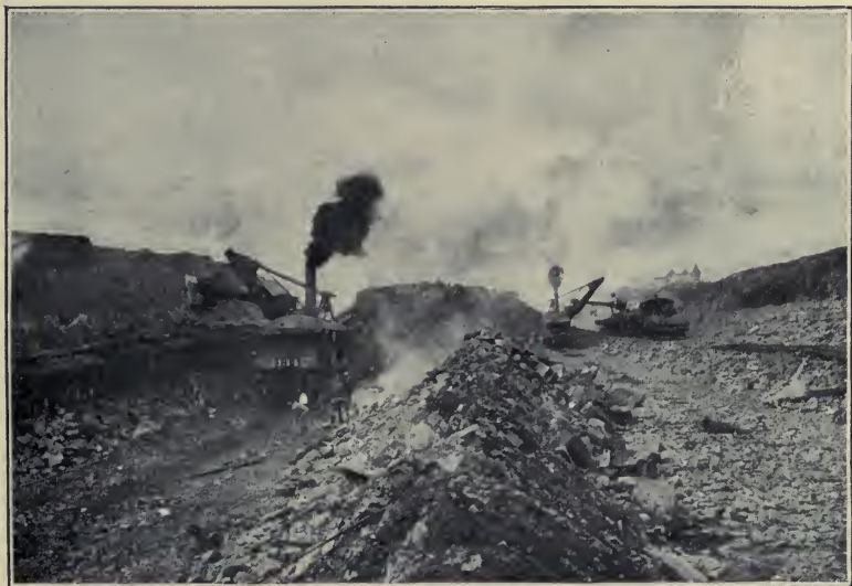
EXCAVATING FOR GATUN LOCKS.
