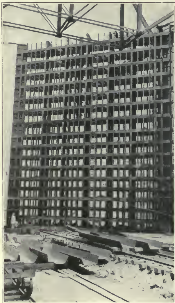
LOCK GATE IN COURSE OF CONSTRUCTION.
