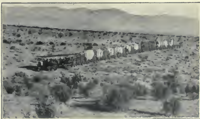
Two 45-h. p. Caterpillars in the Mojave Desert, freighting material for the Los Angeles Aqueduct, one of the engineering wonders of the world.
