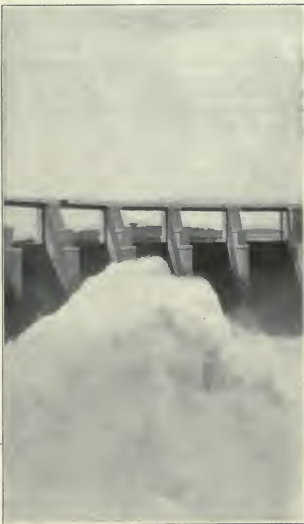
CONE OF LEAPING WATER. GATUN SPILLWAY.
