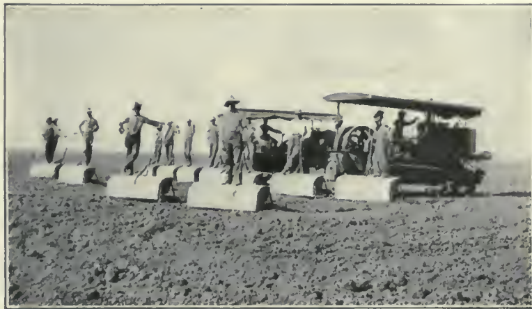
A tractor pulling a battery of scrapers. Grading and leveling land ready for water.
