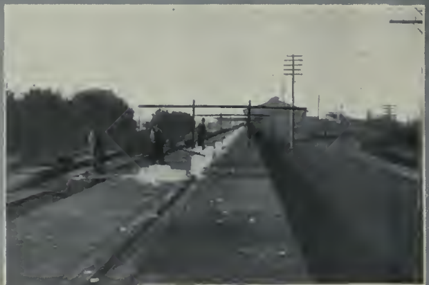
Icing cars at one of the San Joaquin Valley Plants of National Ice and Cold Storage Company of California.
