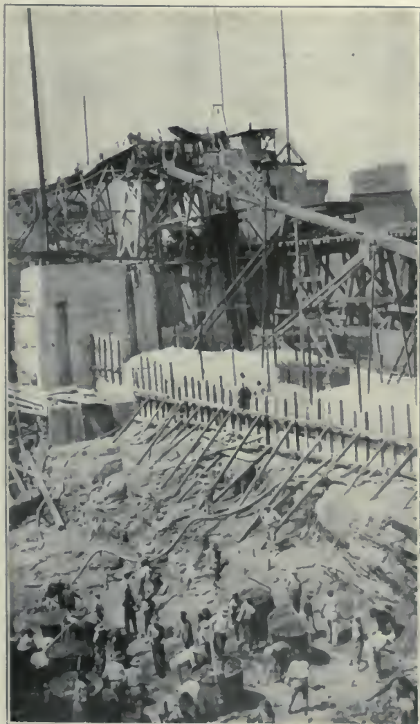
DETAIL OF CONSTRUCTION WORK.
