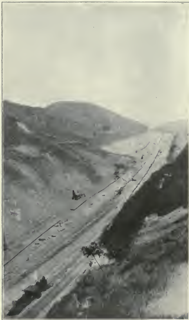
A SLIDE IN THE CULEBRA CUT.
