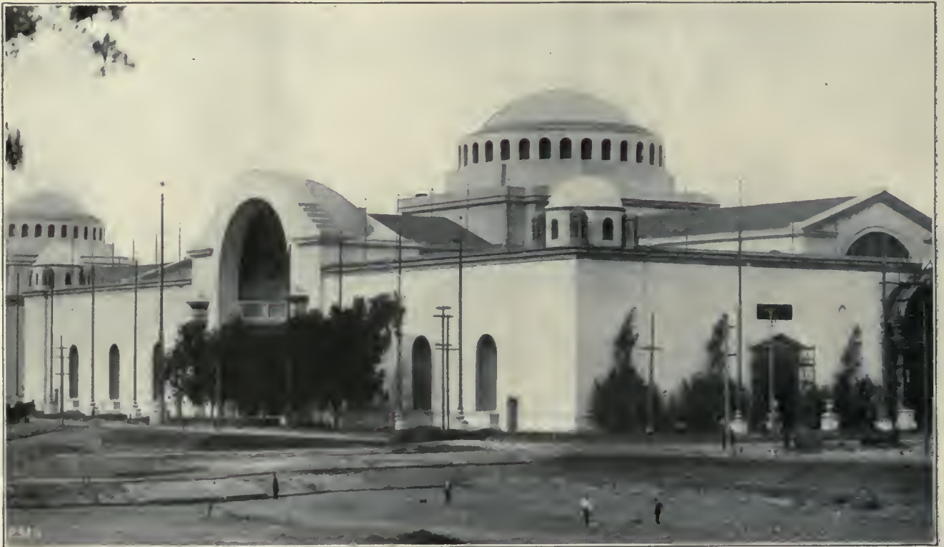
THE PALACE OF EDUCATION, SHOWING THE WESTERN ENTRANCE.
