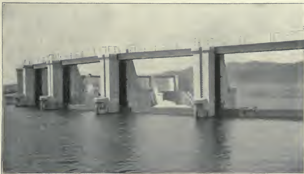
UPPER SIDE OF GATUN SPILLWAY. CONE OF WATER IN DISTANCE.
