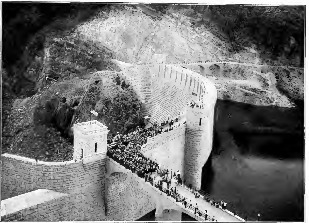
THE ROOSEVELT DAM, SALT RIVER VALLEY, ARIZONA. A GOVERNMENT RECLAMATION PROJECT IRRIGATING, AT PRESENT, 152,000 ACRES.
