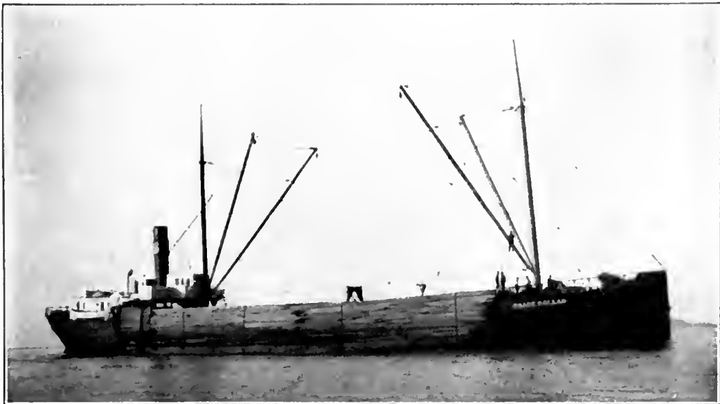
A VESSEL ESPECIALLY DESIGNED FOR TIMBER CARRYING. NOTE THE LENGTH OF CLEAR HULL AND DECK ROOM.
