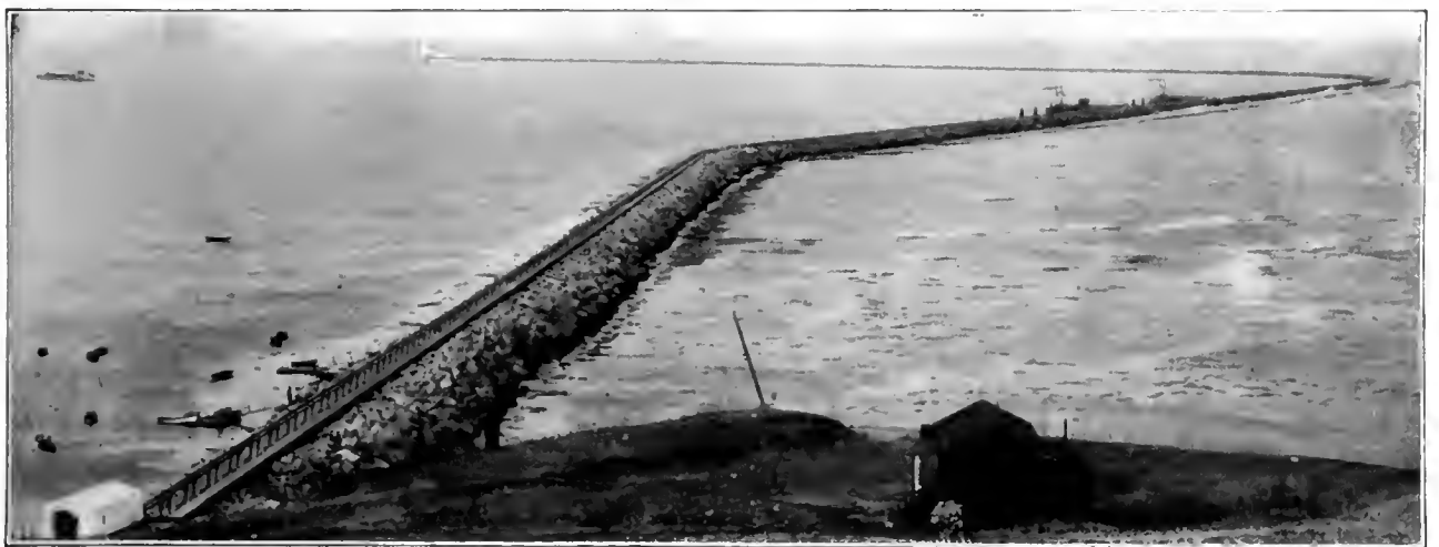
BREAKWATER AT SAN PEDRO—PORT OF LOS ANGELES.
