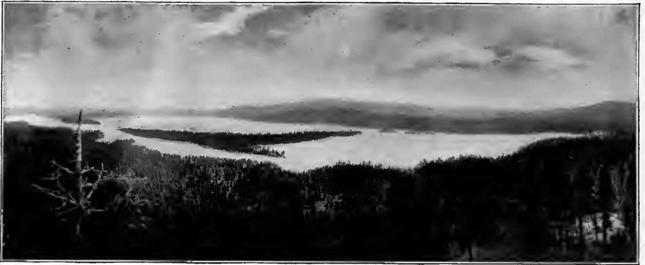
Great Western Power Company's storage reservoir (Lake Almanor) on the North Fork of the Feather River, Plumas County, California—the largest artificial reservoir in the State of California. The lake is over 10 miles in length, has an area of 30 square miles and contains 82,000,000,000 gallons of water, at an elevation of 4,450 feet above sea-level. The equalized river flow resulting from this vast storage reservoir is utilized at the Big Bend Power House where is generated 75,000 continuous electrical horsepower.
