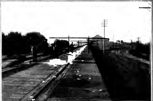
Icing cars at one of the San Joaquin Valley Plants of National Ice and Cold Storage Company of California.
