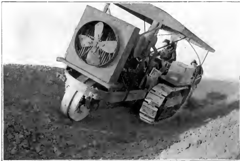
Caterpillar tractor with two-furrow ditching plow building irrigation ditch and levee at the same time.
