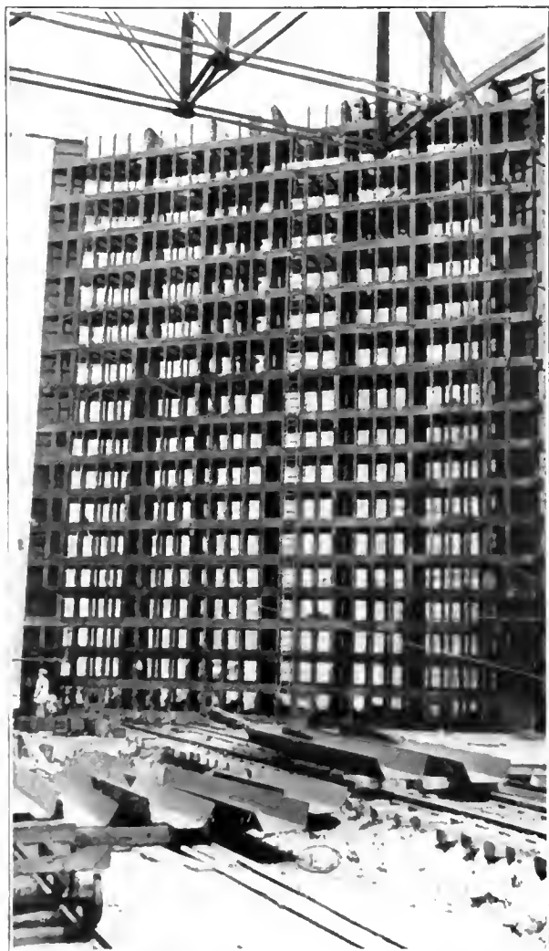
LOCK GATE IN COURSE OF CONSTRUCTION.
