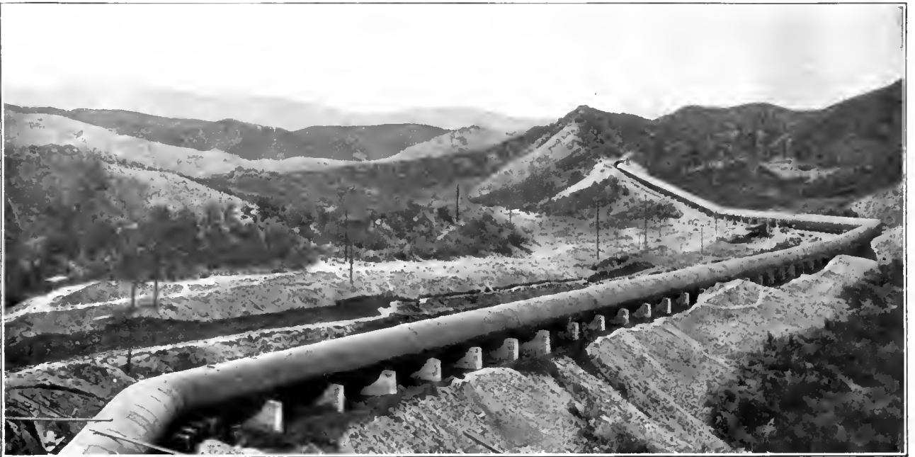
SIPHON ON LOS ANGELES AQUEDUCT. BUILT BY THE CITY. DEADMAN'S CANYON.
