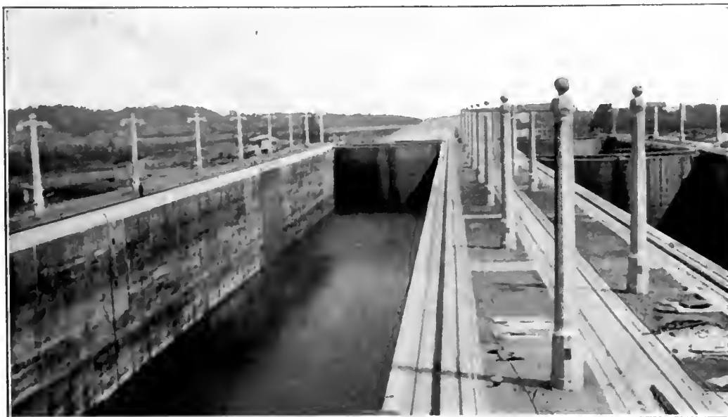
SECOND LOCK LEVEL AT GATUN. CANAL AND OCEAN IN THE DISTANCE.
