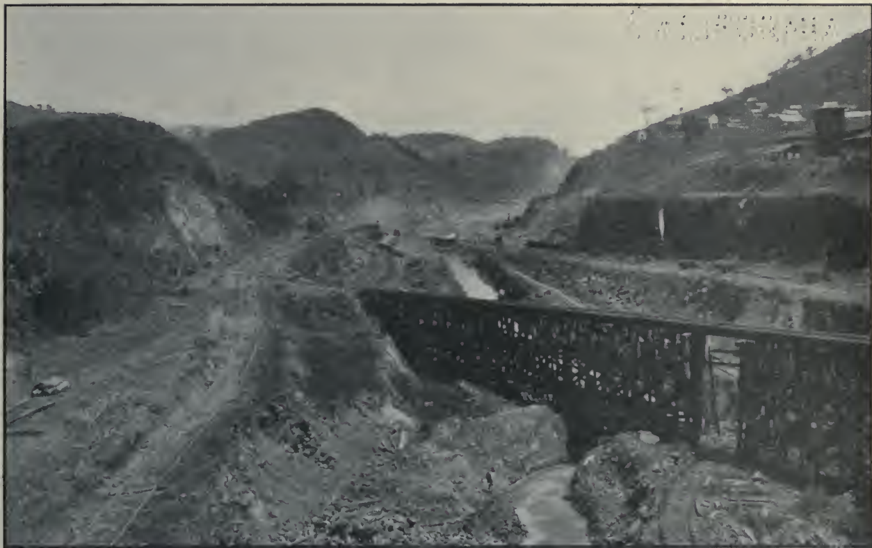
Culobra Cut Looking North from Bridge 57\frac{1}{2} , Near Paraiso. The Train on the Left, Just Beyond the Trestle Bridge, Is on the Completed Bottom of the Canal, Elevation +40. Photographed June, 1912.
