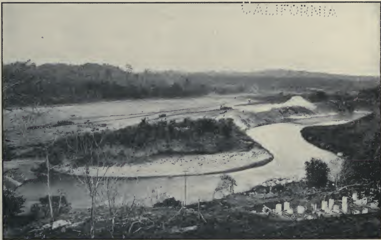
Channel Excavated at San Pablo During Dry Season, 1912. This Channel Is Completed and Is 800 Feet Wide, With Bottom Elevation at +40.
