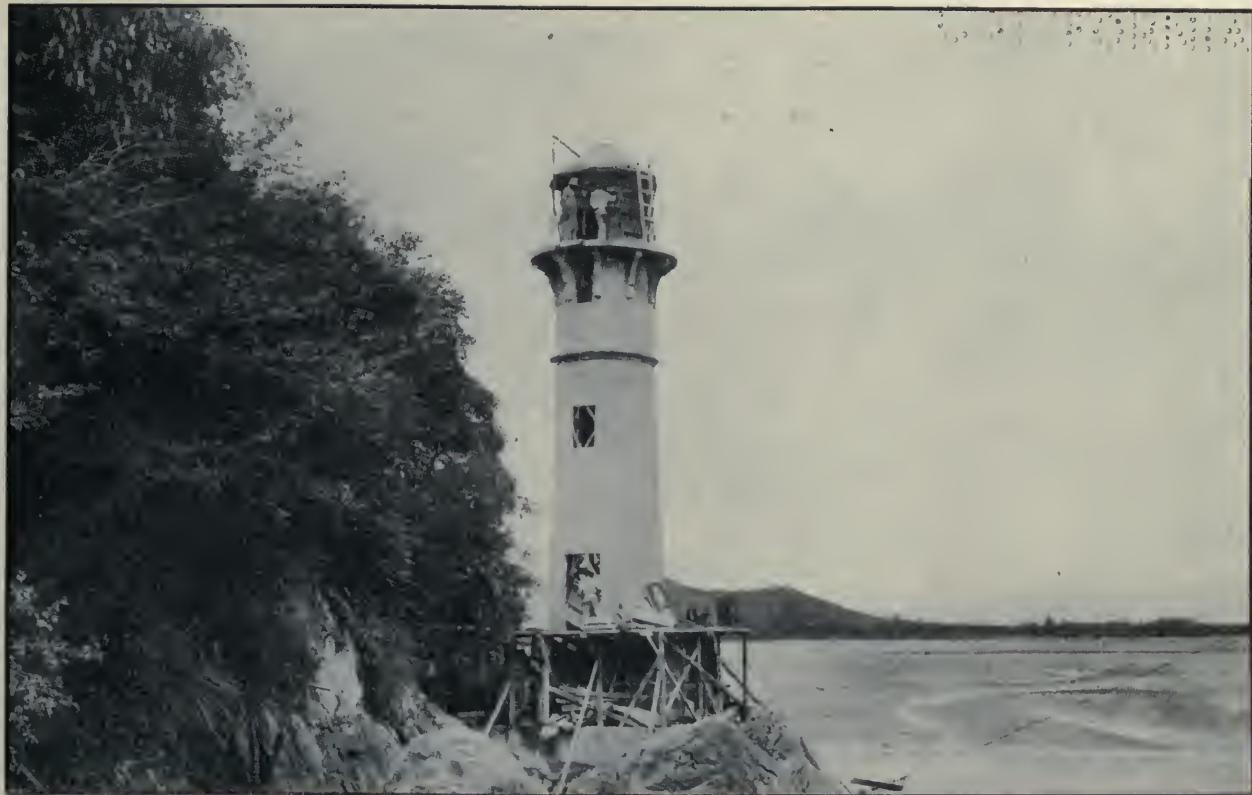
Rear Tower, Range 9-11, Pacific Entrance, Looking Northwest. This Is One of the Efficient Range Lights that Will Make the Navigation of the Canal Safe and Easy, Night and Day.
