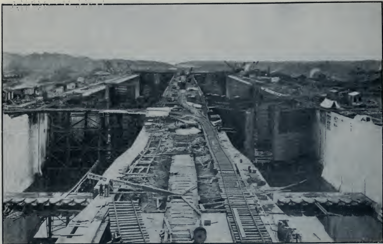
Gatun Upper Locks, Looking North from Lighthouse, as They Appeared July 2, 1912. The Three Pairs of Locks at Gatun Have a Combined Lift of 85 feet.
