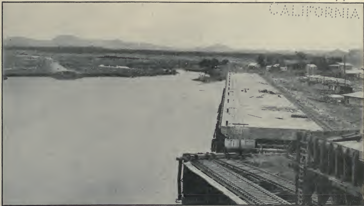
Balboa—Lumber Dock of Reinforced Concrete, Looking Northeast. June, 1912. This Pacific Port at the Southwestern End of the Canal Will Benefit Largely from Its Construction.
