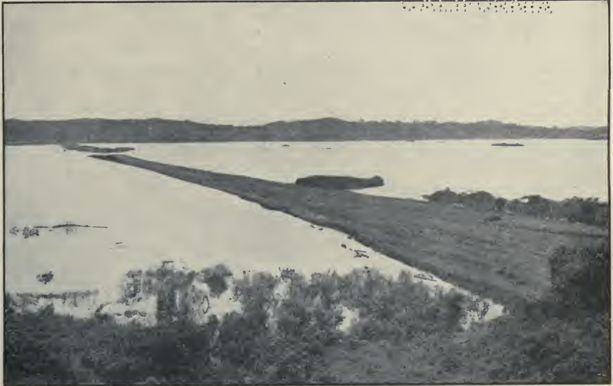
Embankment of Old Panama Railroad Excavated Down to +35 in April and May, 1912.
