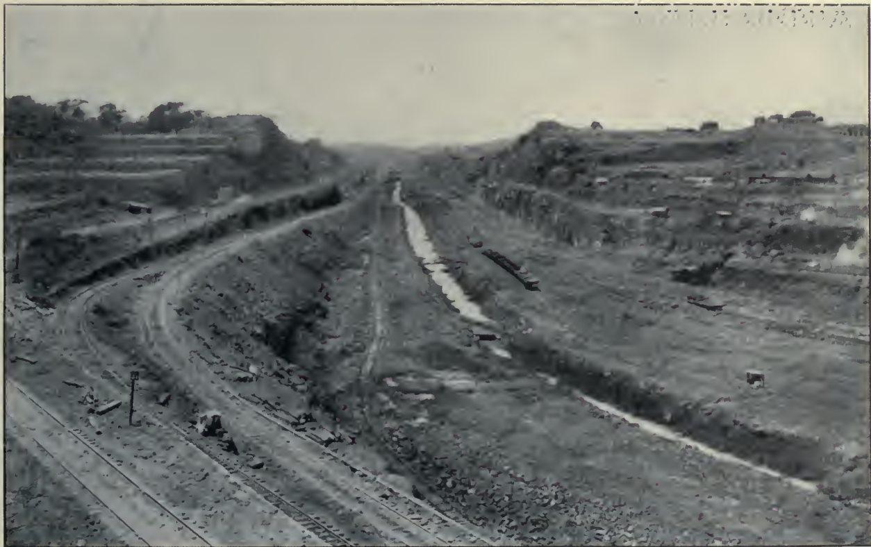
Culebra Cut Looking South from Bend in East Bank Near Gamboa. The Train and Shovel Are Standing on the Bottom of the Cut. The Water in the Drainage Channel Is About 10 Feet Below the Bottom of the Canal, or at Elevation +30. Photographed June, 1912.
