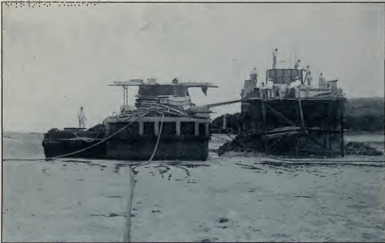
Front Tower, Range 9-11, Pacific Entrance Looking Southeast. Photographed November 7, 1911, and Showing the Reinforced Concrete Construction of the Lighthouses.
