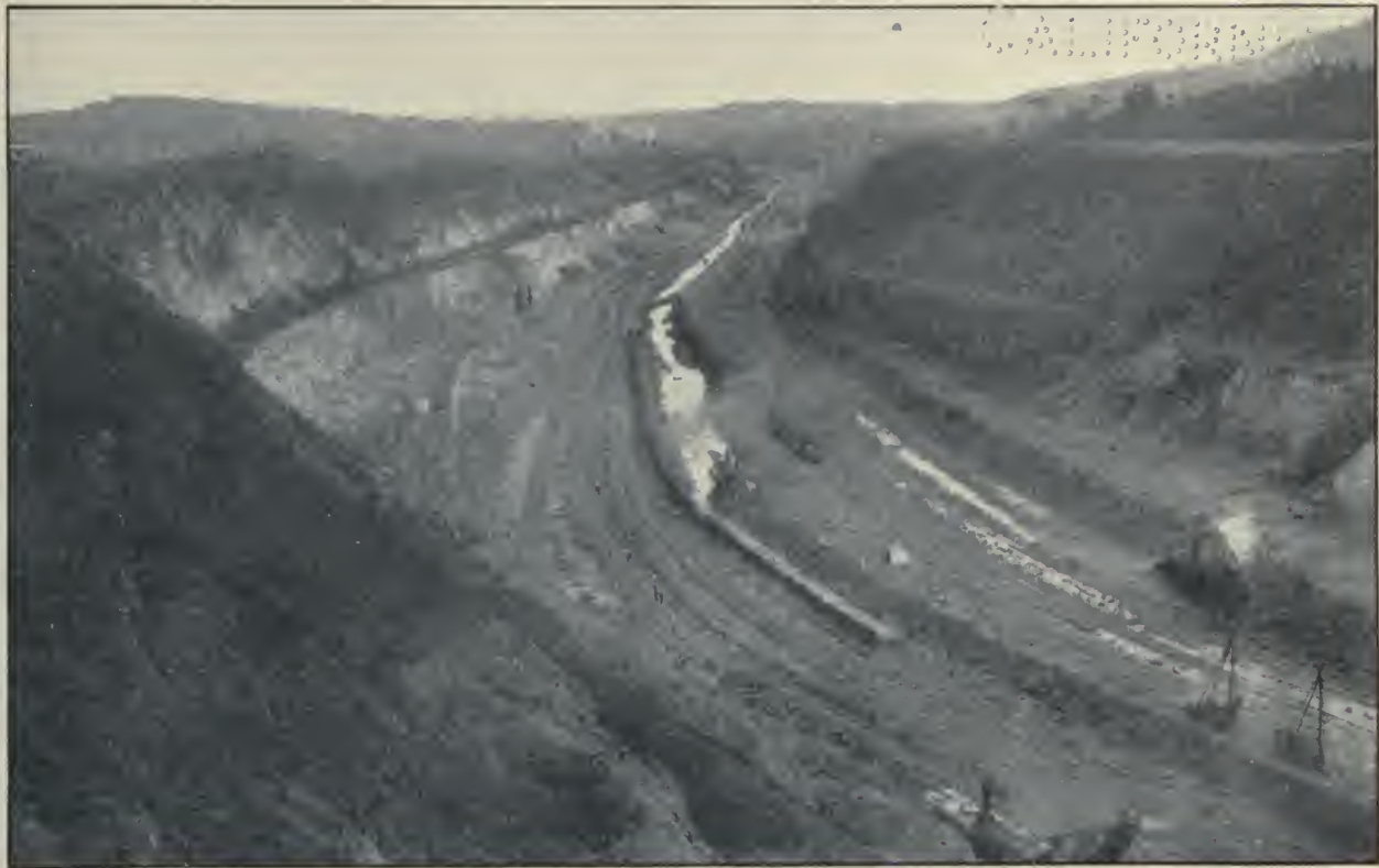
Culebra Cut Looking North from Cunette. The Two Shovels Shown in the Foreground Are Working on the Bottom, Elevation +40. The Water Standing in the Center Drainage Channel Is About 6 Feet Below the Bottom, Elevation +34. Photographed in June, 1912.
