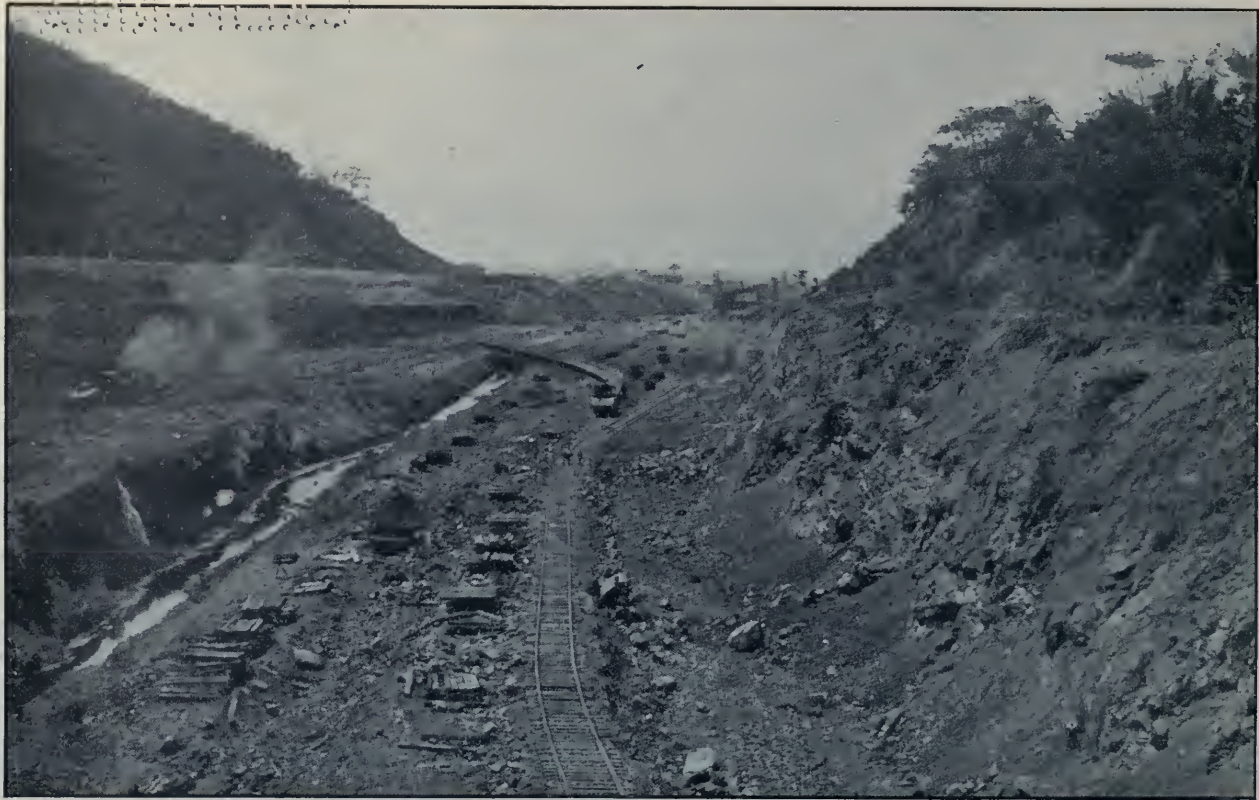
Culebra Cut, South End, Looking South from Bridge 57½ and Showing the Partly Completed Anchorage Basin North of Pedro Miguel Lock. Train Is on Completed Bottom of Canal, Elevation +40. Photographed June, 1912.
