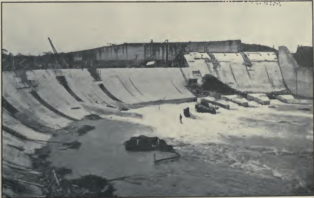
Gatun Spillway Looking Southwest, Showing Downstream Face of Ogee Dam, as it Appeared June 6, 1912.
