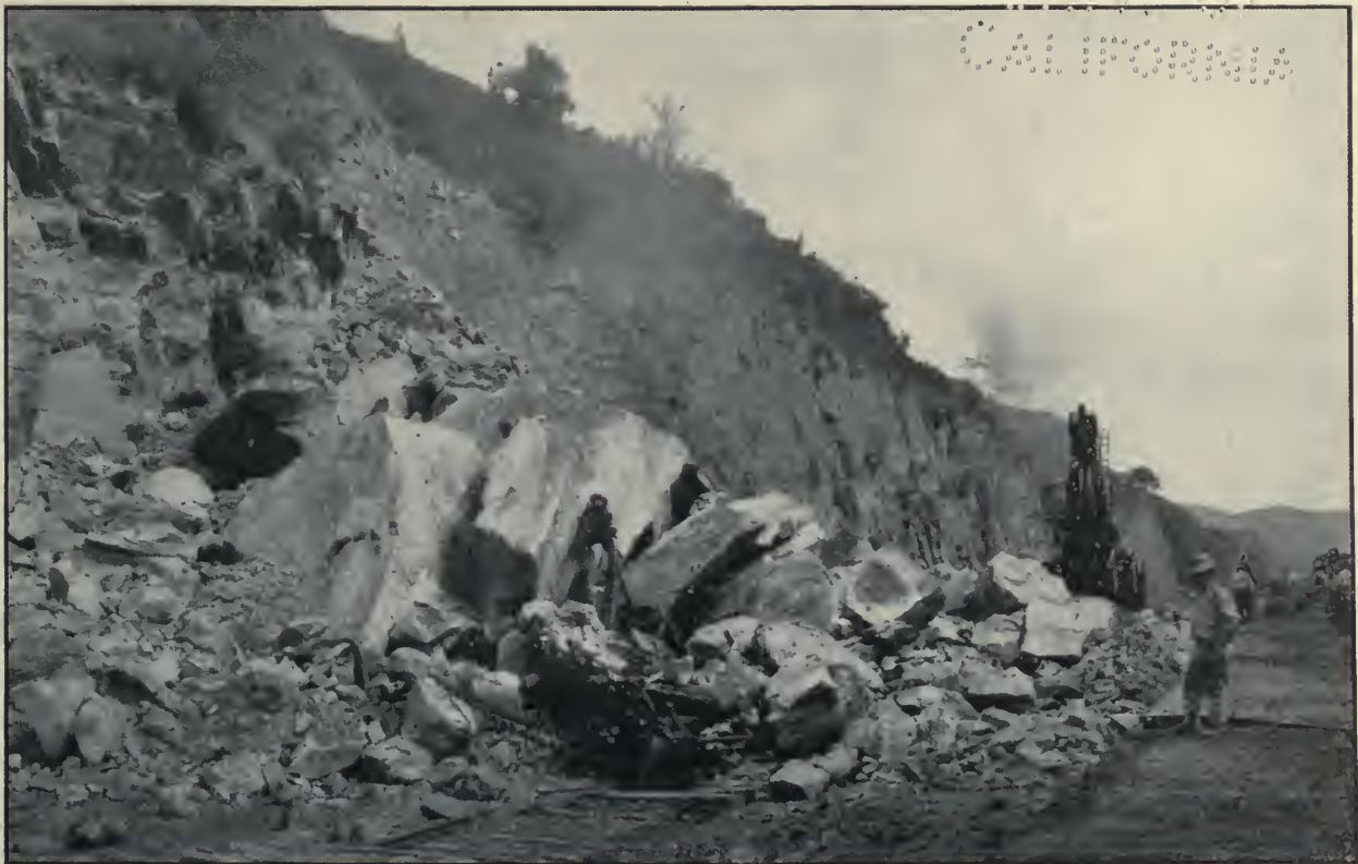
Steam Shovel 218 Buried Under Fall of Rock, West Side of Canal, Near Las Cascadas. This Shovel Was Working on the Bottom of the Canal When Destroyed, May 31, 1912.
