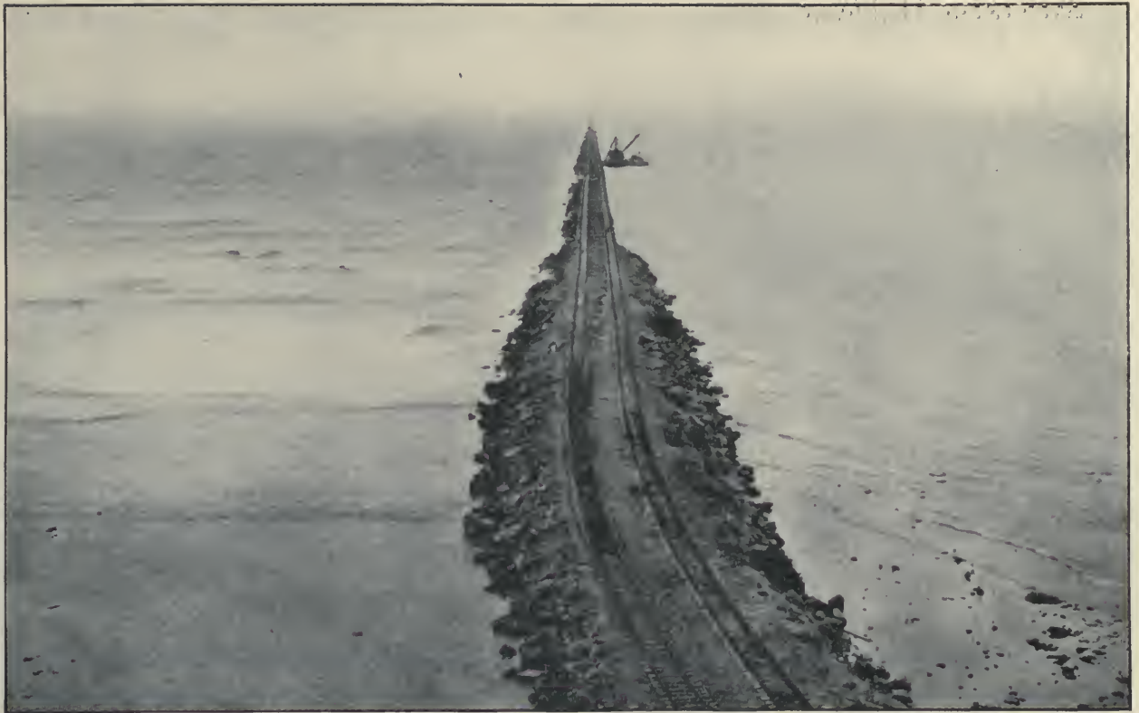
West Breakwater, Looking Seaward from Toro Point, Showing Dredge at Work Placing Rock on Face of Breakwater. Photographed June, 1912.
