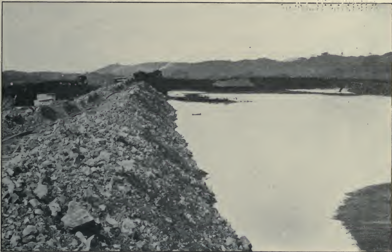
Gatun Dam, West Section of Dam Looking West, Showing Progress of Hydraulic Fill, June 12, 1912. This Great Dam Is Nearly 1\frac{1}{2} Miles Long and About \frac{1}{2} Mile Wide at Its Base.
