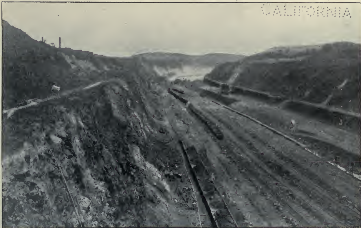
Culebra Cut, Looking North from Empire Suspension Bridge. The Nearest Shovel Shown, in the Lowest Cut, Is Working About 12 Feet Above the Bottom, or at Elevation +52. The Photograph Was Taken in May, 1912.
