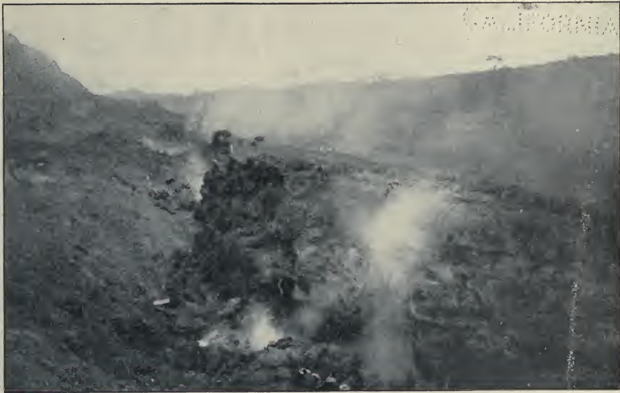
Heated Material on the West Side of the Canal, 350 Yards North of Culebra y. Extent of Heated Material 500' x 25' x 20'. Photographed February 16, 1912.
