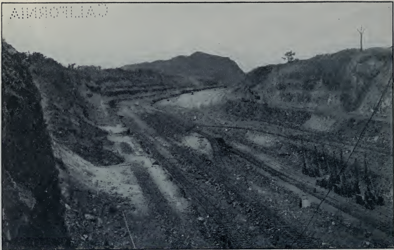
Culebra Cut, Looking South from Empire Suspension Bridge. The Group of Well Drills in the Middle of the Canal Is About 27 Feet Above the Bottom, or at Elevation +67, Photographed May, 1912.
