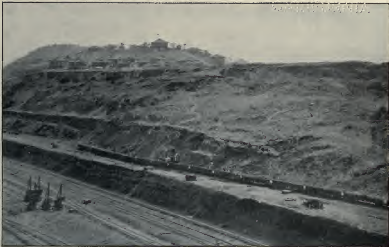
Slide of Stratified Rock, West Bank of Canal, Culebra-on-the-Dump, Looking Toward Culebra. Slide Involves About 1,000,000 Cubic Yards and Moved About 3 Feet Per Day on a Slope of 1 Vertical to 7 Horizontal. The Train Is Standing at Elevation +95. Photographed February, 1912.
