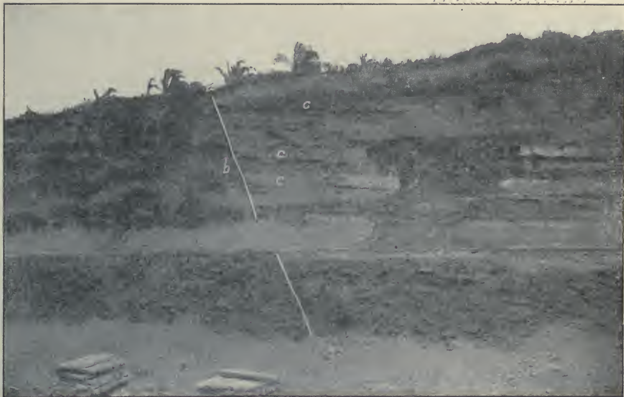
"A" Fault Plane. "B" Crushed and Sheared Zone of Rock. "C" Stronger Rocks, Beds of Limy Sandstone. This Fault Was the Chief Cause of the Big Slide on the West (Opposite) Side of the Canal Near Lirio.
