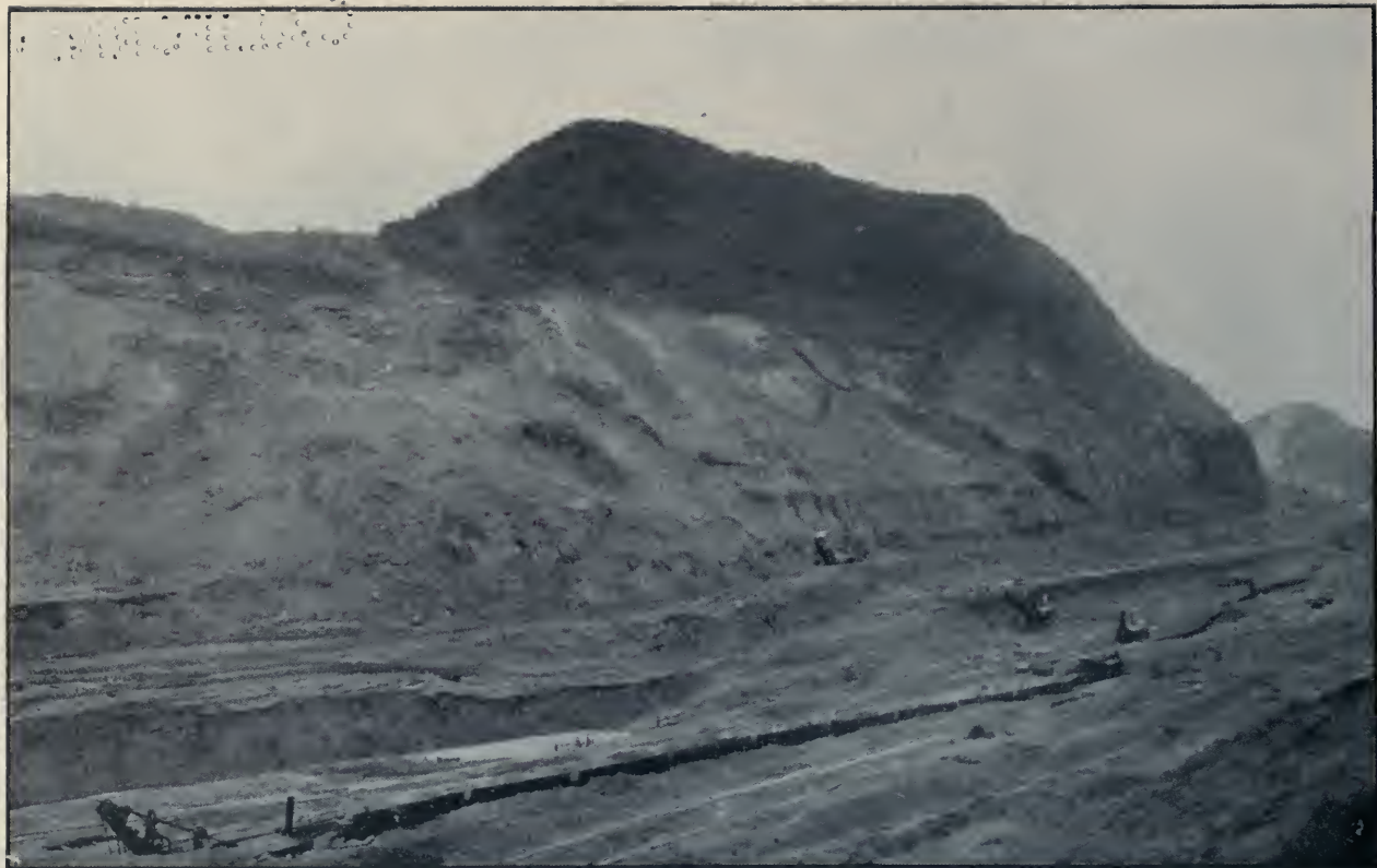
Culobra Cut, Culobra. Break in East Bank of Canal. Amount of Material Involved, 320,000 Cubic Yards. The Train Shown in Foreground Is About 35 Feet Above the Bottom, or at Elevation +75. Photographed February 11, 1912.
