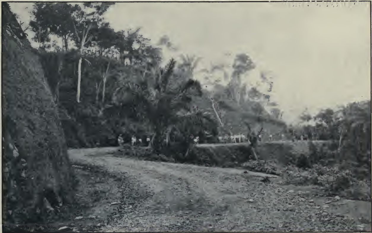
Empire-Chorrera 16-Foot Macadam Road Under Construction with Zone Prison Labor, as It Appeared August 29, 1912.
