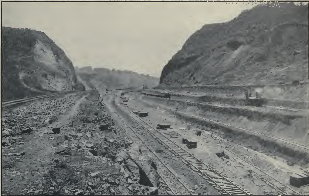
Culebra Cut Looking South from Cunette. The Two Shovels Shown in the Foreground Are Working on the Bottom of the Canal, Elevation +40. Photographed in May, 1912.
