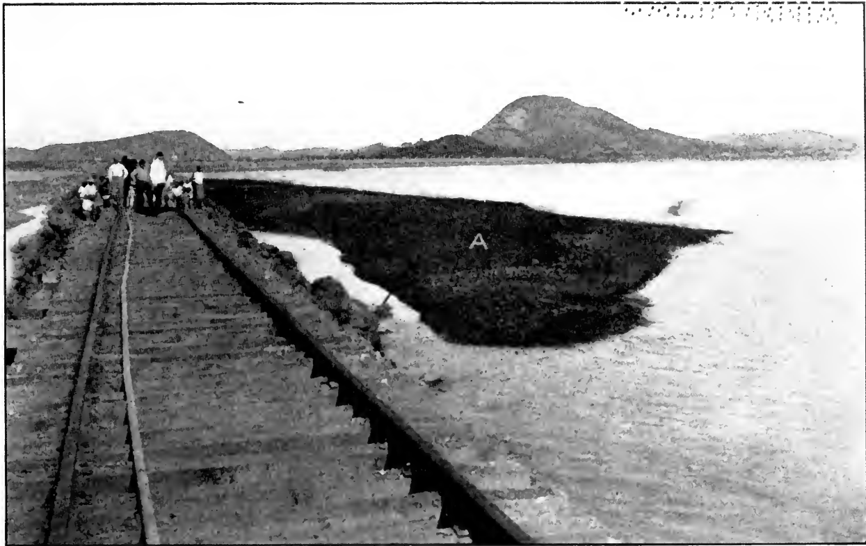
South End of Naos Island Dump, 4,000 Feet from Island. Center at "A" is 75 Feet from Track and 25 Feet Above the Original Bottom. Elevation of Trestle, +14. Photographed December, 1911.
