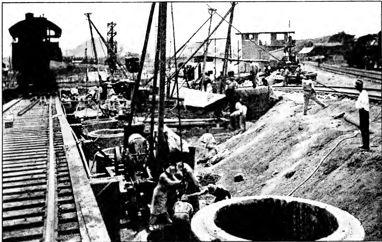
Mirafleres Locks. Sinking Caissons for Foundation of North Approach Wall, Looking North, June 14, 1912.
