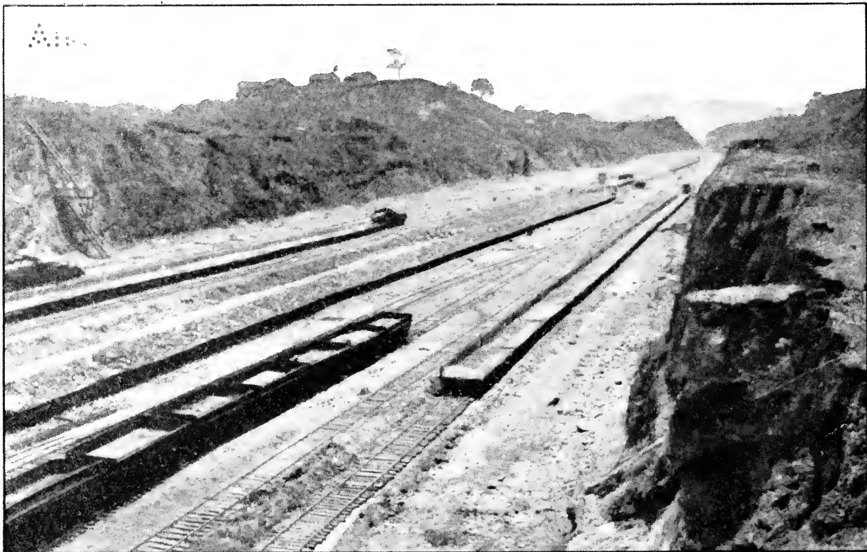
Culebra Cut Looking North from Las Cascadas. All Trains Are Standing on the Bottom of the Cut, Elevation +40. Photographed May, 1912.
