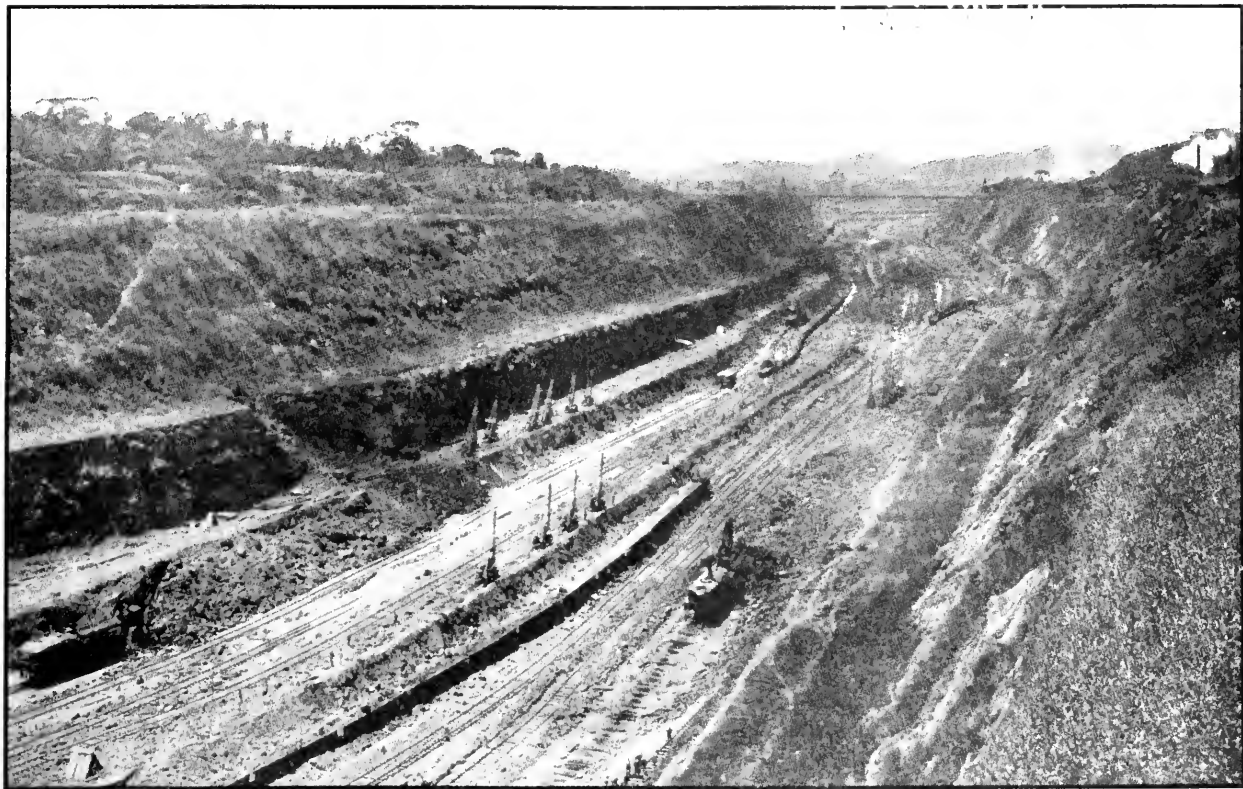
Culebra Cut, Looking North from a Point South of Contractor's Hill, Showing Quiescent State of the Great Cucaracha Slide on Right Bank. Photographed May, 1912.
