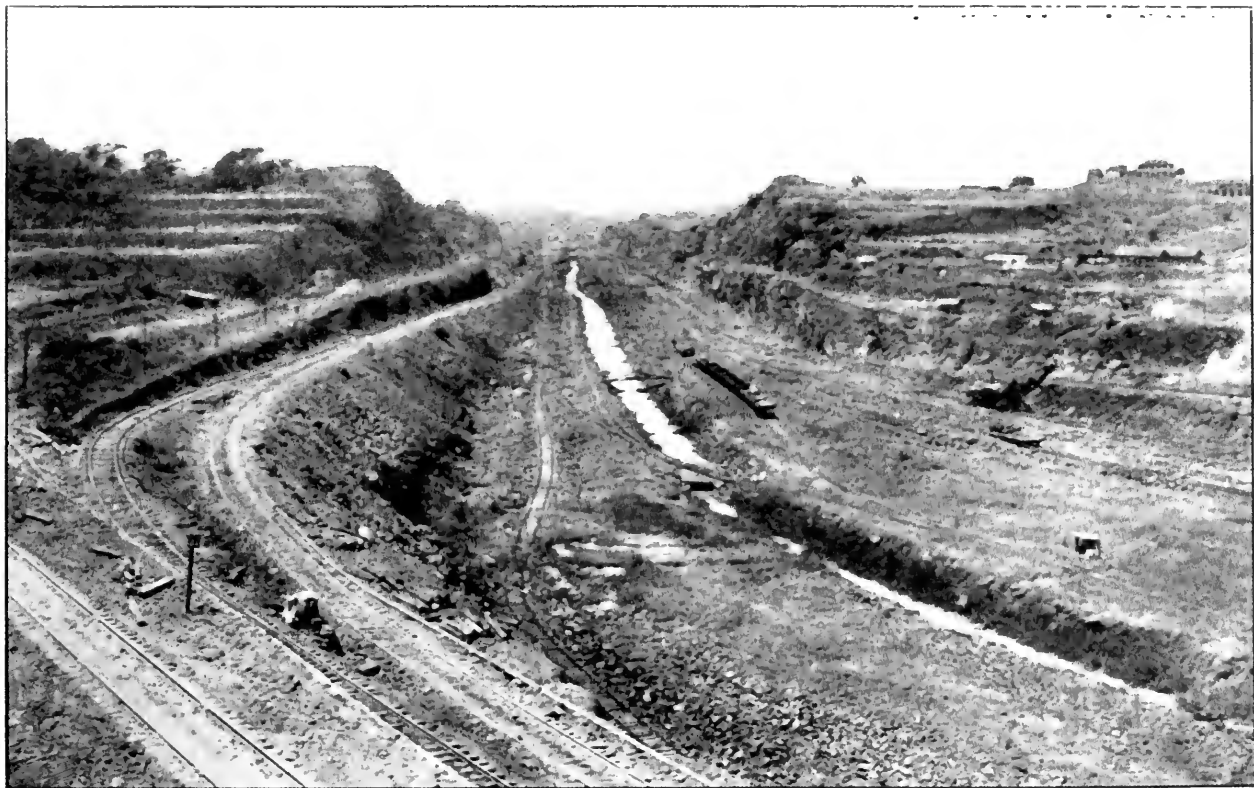
Culebra Cut Looking South from Bend in East Bank Near Gamboa. The Train and Shovel Are Standing on the Bottom of the Cut. The Water in the Drainage Channel Is About 10 Feet Below the Bottom of the Canal, or at Elevation +30. Photographed June, 1912.
