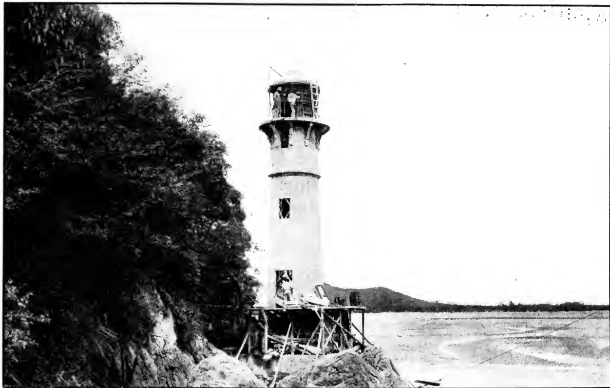
Rear Tower, Range 9-11, Pacific Entrance, Looking Northwest. This Is One of the Efficient Range Lights that Will Make the Navigation of the Canal Safe and Easy, Night and Day.
