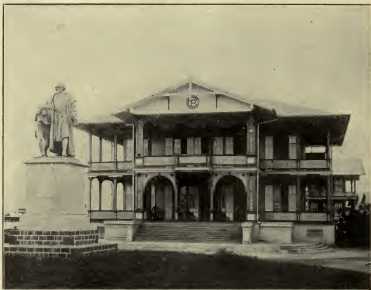
LESSEPS VILLA (NOW CANAL OFFICES) AND STATUE OF COLUMBUS, CRISTOBAL, CANAL ZONE.
