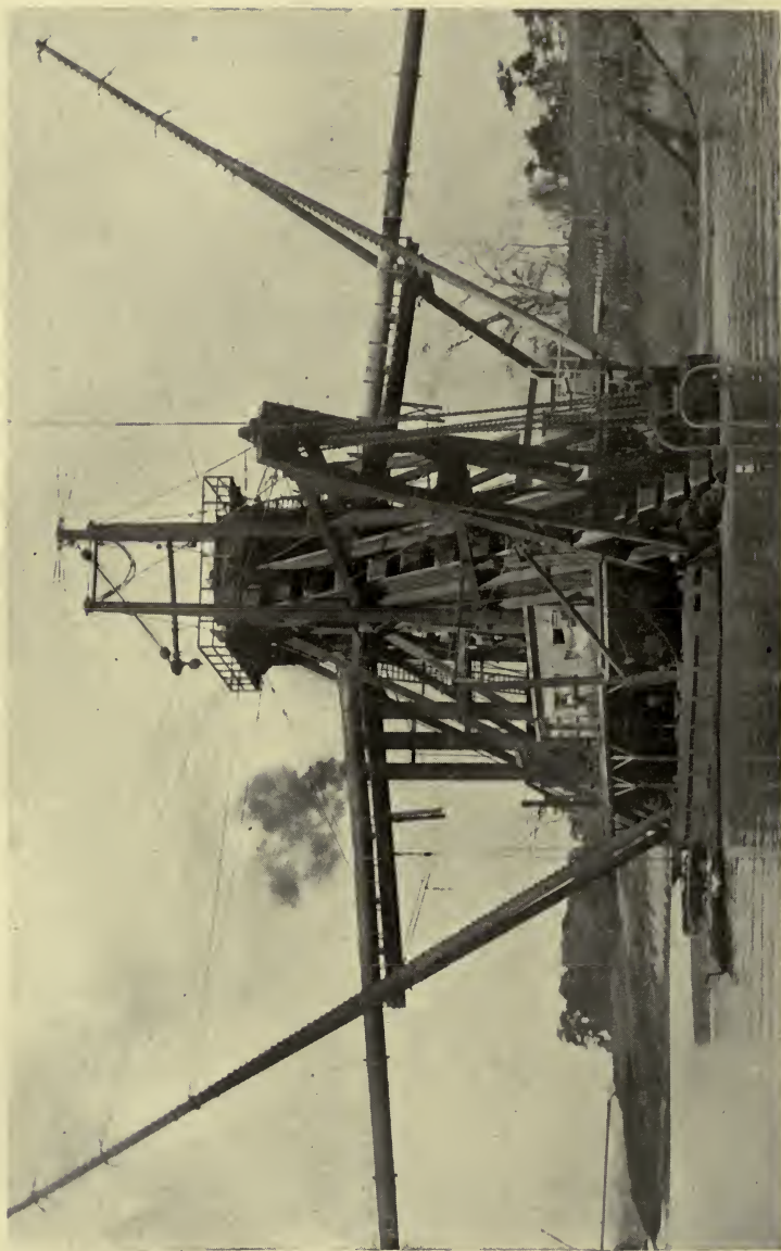
A SLAVEN DREDGE AT WORK (ABOUT 1885) ON THE FRENCH CANAL.
