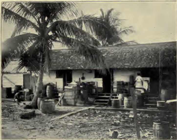
FORMER STREET-SCENE, COLON.
