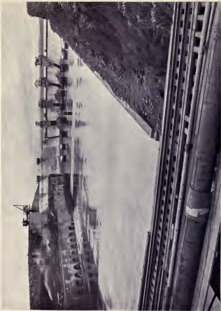
THE SPILLWAY AT GATUN, SHOWING THE RISING SURFACE OF GATUN LAKE IN THE DISTANCE, SEPTEMBER 7, 1912.
