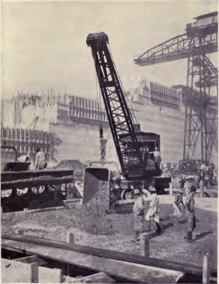
DUMPING CONCRETE FOR THE WALLS OF THE PEDRO MIGUEL LOCKS, NOVEMBER, 1910.
