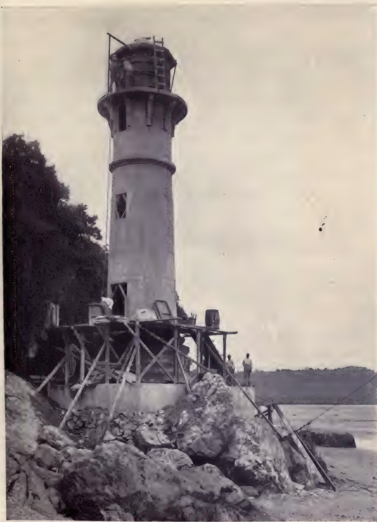
BUILDING A LIGHTHOUSE ON THE EDGE OF THE JUNGLE.
