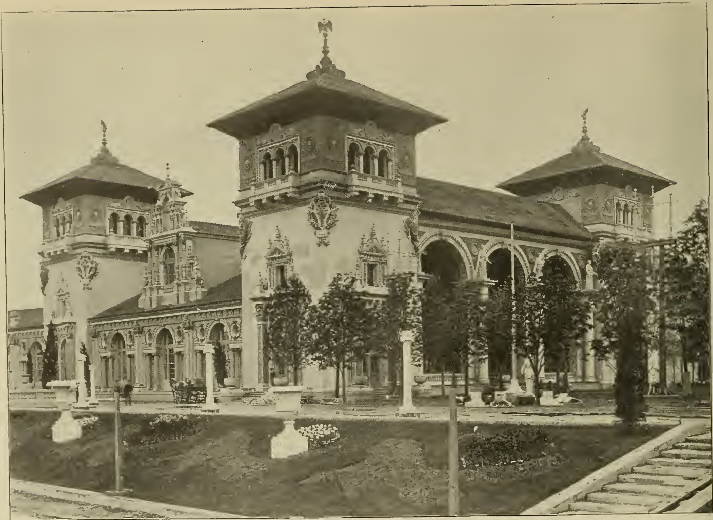
GRAPHIC ARTS BUILDING, 150 ft. square
