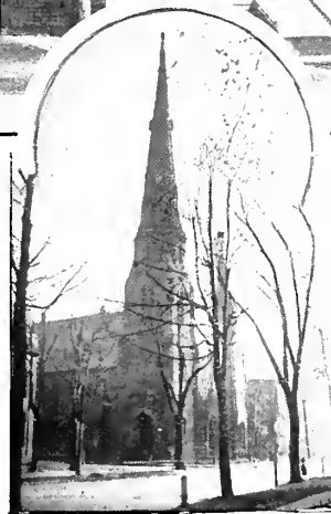
DELAWARE AVENUE ~ METHODIST CHURCH
