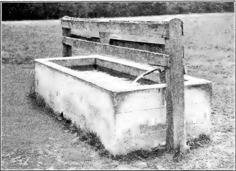
FIGURE 10.—Type of sanitary watering trough
