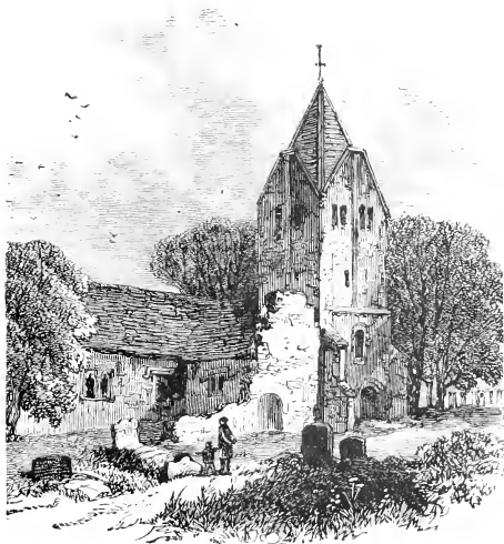
Saxon tower, Sompting Church, Sussex.
