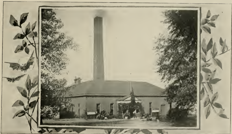
WATER WORKS AND ELECTRIC LIGHT PLANT
