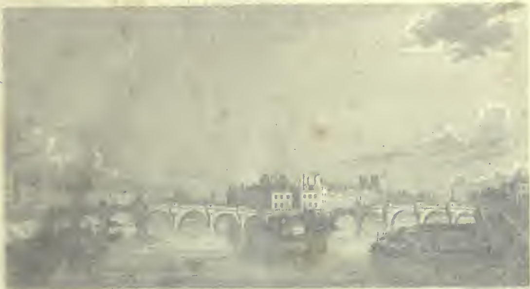
BRIDGE OVER THE RIVER AT ST. LOUIS.
