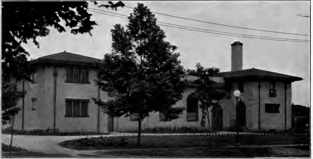
PLATE No. 207. RHODIUS PARK COMMUNITY HOUSE, INDIANAPOLIS
