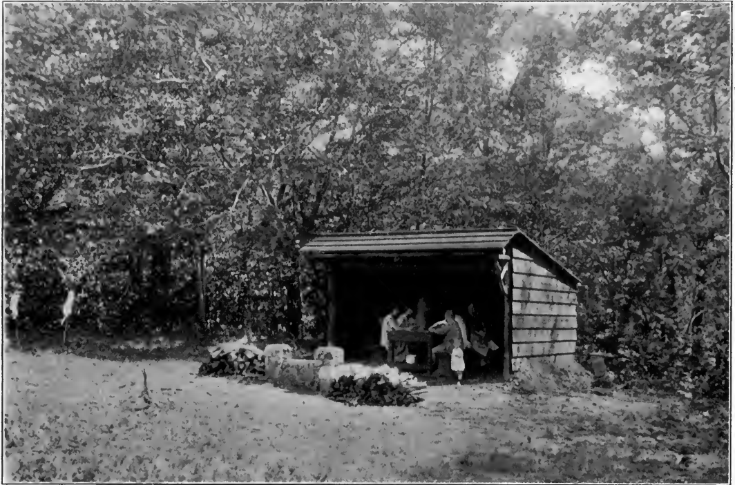
PLATE No. 184. A TYPE OF ADIRONDACK SHELTER
