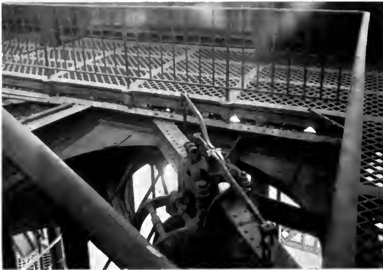
THE MECHANISM FOR STRIKING BIG BEN.
