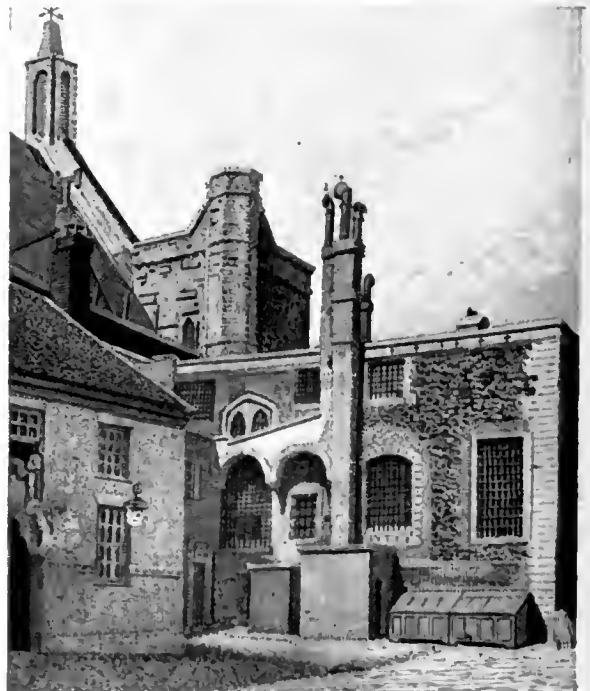
THE SPEAKER'S COURTYARD, FROM THE SOUTH-EAST. Another back view of the Speaker's residence in the old Palace of Westminster.
