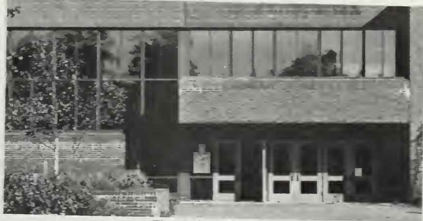
Where do these doors lead?
