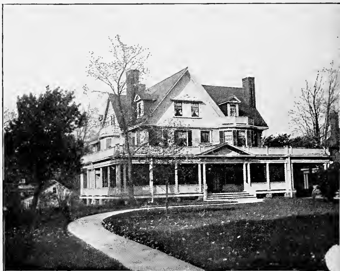
RESIDENCE OF EDWARD P. ALLING, EAST ORANGE.
