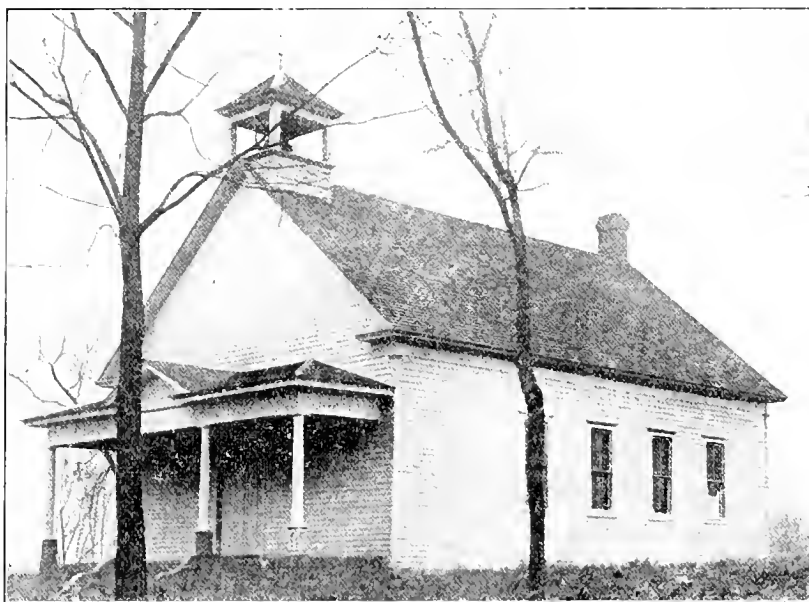
HICKORY SPRINGS, FRANKLIN TOWNSHIP.
