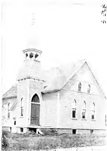
METHODIST EPISCOPAL CHURCH. SEATON
