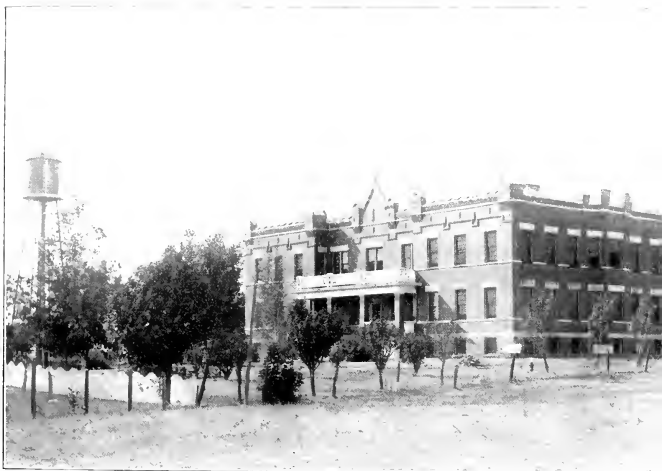
MERCER COUNTY FARM AND HOME
