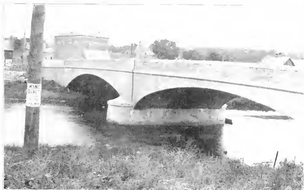
CONCRETE BRIDGE OVER UPPER IOWA RIVER, DECORAH
