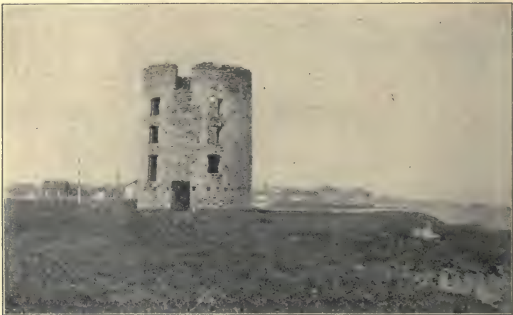
Martello Tower of Refuge in Time of Indian Wars—Three Rivers.
