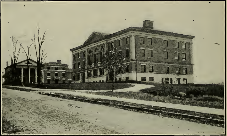
STATE NORMAL SCHOOL BUILDINGS, NORTH ADAMS
