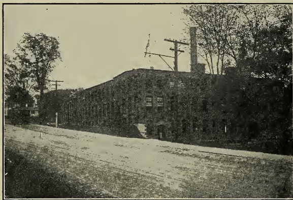
CRANE'S GOVERNMENT MILL, PITTSFIELD
