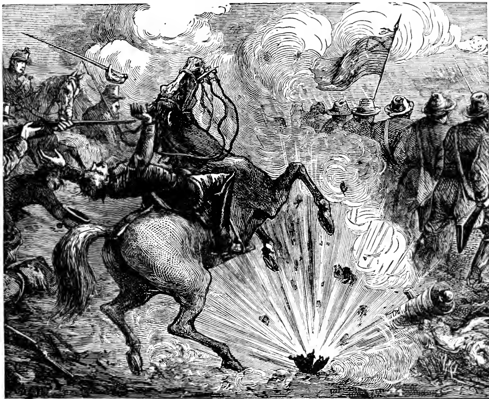
PURIFIED THROUGH FIRE.
