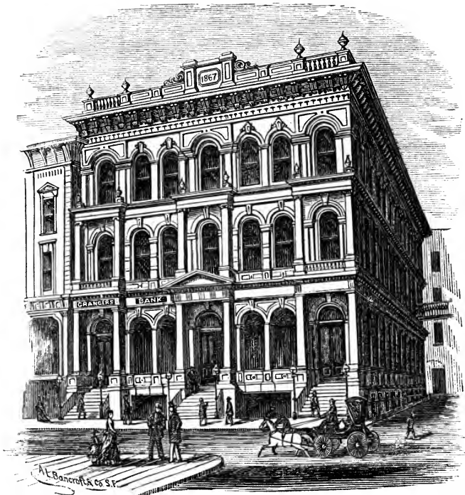
THE GRANGERS' BANK; Offices of Fire Insurance Association and Executive Committee, Corner California and Leidesdorff Streets, San Francisco.
