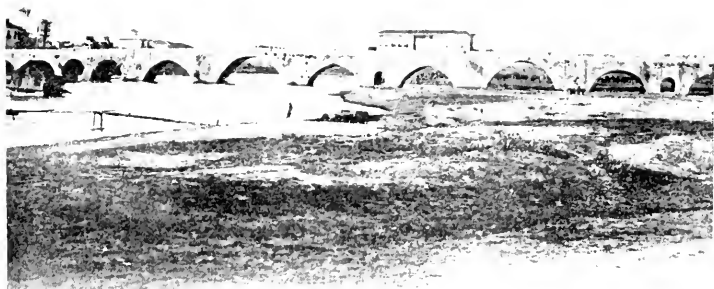
FIG. 11.—The Bridge over the Saros at Adana (Mrs. Christie of Tarsus). To face p. 176. See p. 274.
