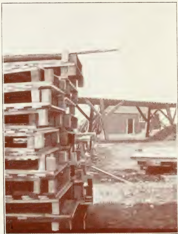
FIG. 40.—Empty Palettes for Air-drying Peat.
