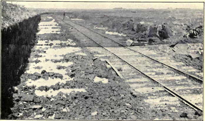
Working Trench at Ökaer, Denmark.
