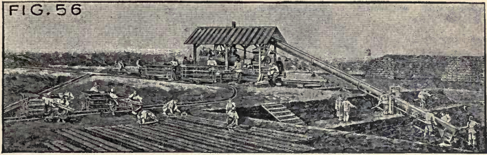
FIG. 56—Schlickeysen's Peat Machine with end elevator.
