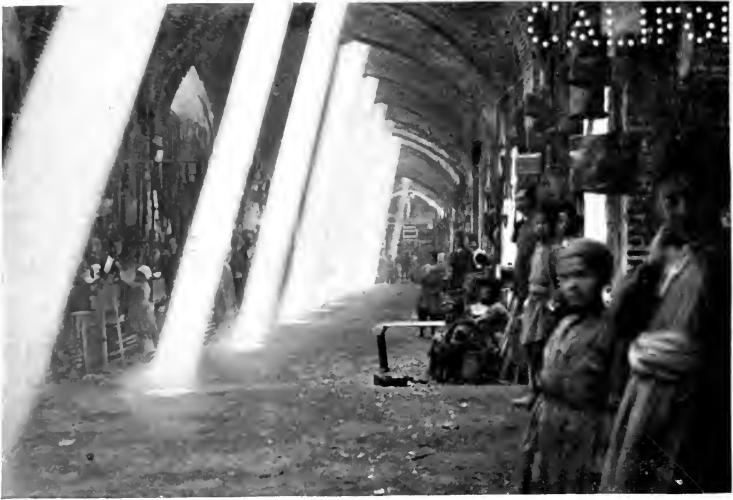
The Bazaar. Showing how the light comes through the roof.
