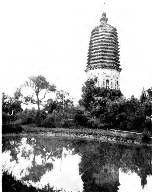
Lama Tower 1,600 years old, Liaoyang
