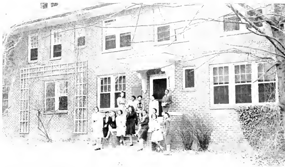
The Tuttle Building, Side View
