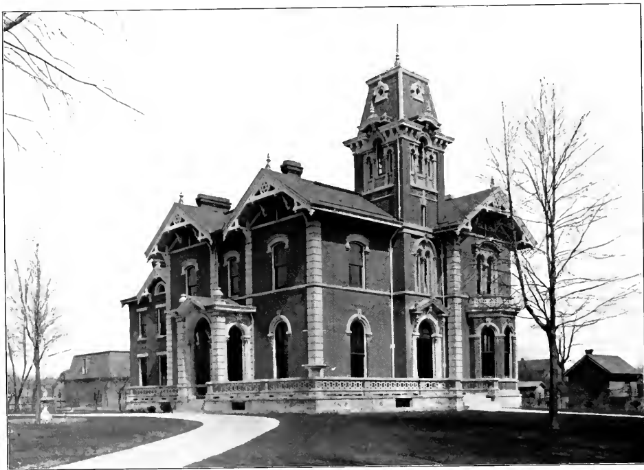
Residence of Hon. Francis T. Roots
