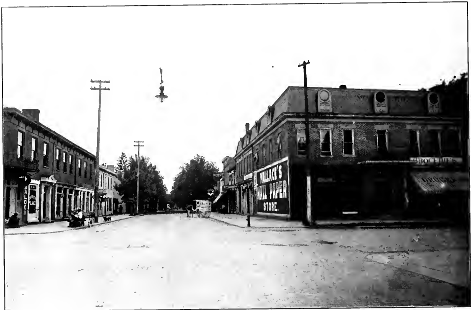
Looking South on Central Avenue from Fourth Street
