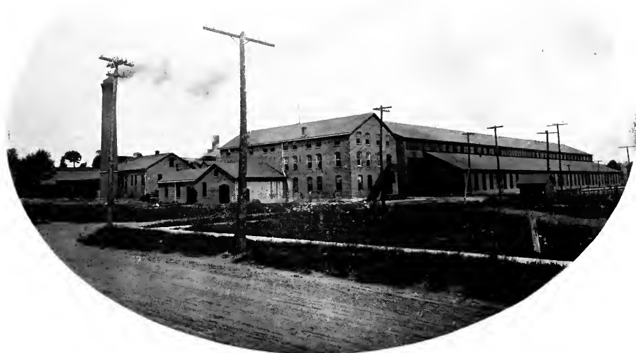
Connersville Blower Co.—Side View of Plant
