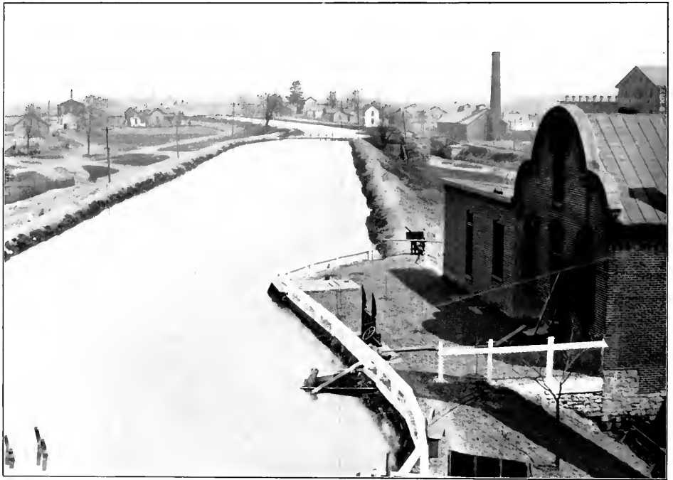
The Hydraulic and Water Works
