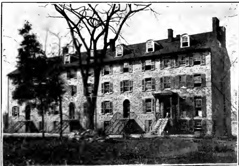
DICKINSON COLLEGE CARLISLE, PA. EAST BUILDING.
