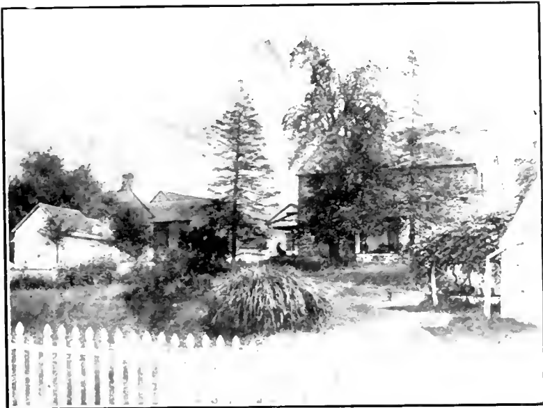
YOST HOMESTEAD IN WHITPAIN, MONTGOMERY COUNTY, PA.
