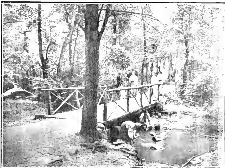
CROSSING THE FOOT BRIDGE.
