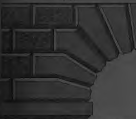
No. 4 represents half of another arch with venous forming an eccentric curve from that of the right column, or else a pointed arch, while the intrados form a concave surface.
