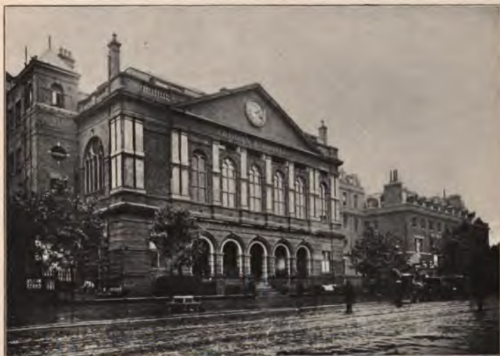
LONDON HOSPITAL, MILE END ROAD.
