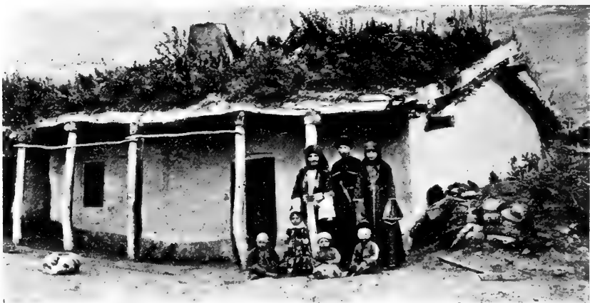
Fig. 47. A Karachai House. The Karachai, a Cis-Caucasian Turkic tribe live on the upper course of the Kuban River. The dwelling is made of clay-covered willows.
