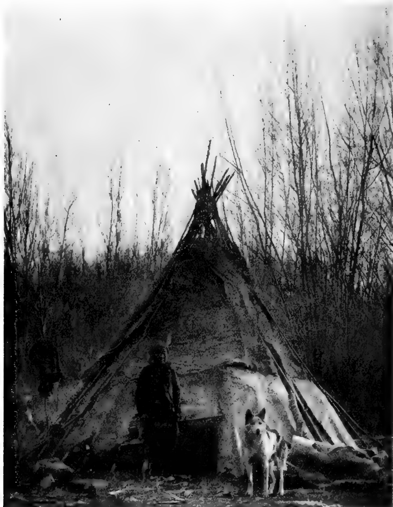
Fig. 37. Conical Summer Tent of the Upper Kolyma Yukaghir. The cover consists of three separate strips of soft tanned reindeer skin fastened to the frame.
