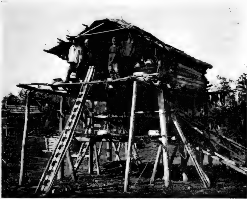
Fig. 52. A Kamchadal Storehouse which also serves as a Summer Dwelling. Such houses have two or three floors and in the upper one food is stored out of reach of the dogs. The lower floors are used for storing clothes and household belongings.
