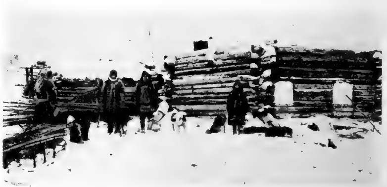
Fig. 45. A Flat-Roofed Blockhouse of the Upper Kolyma Yukaghir which serves as a Winter Dwelling. The windows are covered with thick panes of river ice.
