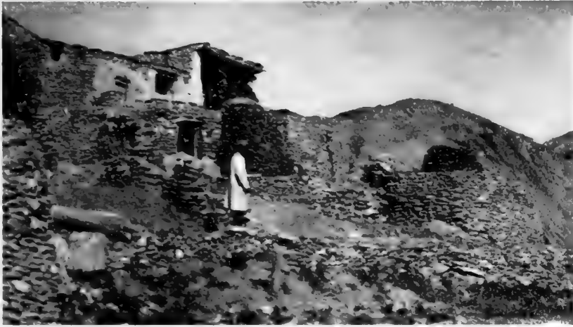
Fig. 51. Galcha Summer Dwelling in the Mountains of the Yagnob, a Tributary of the Zarafshan River. The two-storied house is built of cobbles cemented with clay, the lower for cattle, the upper for the family.
