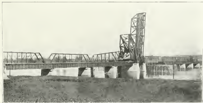
NEW BRIDGE ACROSS THE ILLINOIS RIVER
