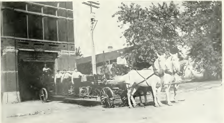
FIRE DEPARTMENT, FIRE TRUCK
