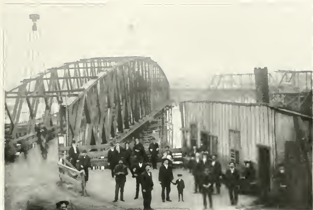
SCENE AT COLE BRIDGE, FOOT OF BRIDGE STREET, JUST BEFORE BRIDGE WAS TORN DOWN IN 1908 FOR NEW STRUCTURE The bridge "crowd" say "good-bye"
