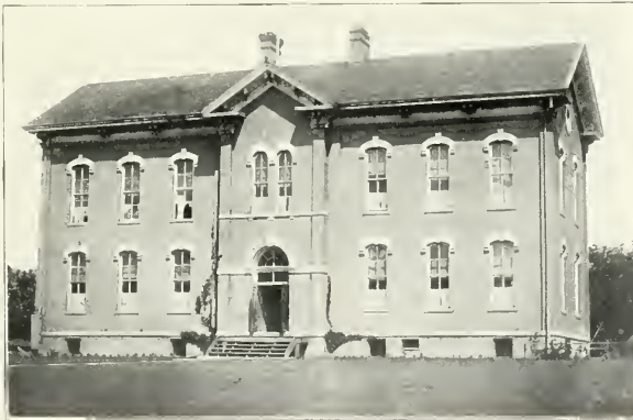
OLD FIFTH WARD SCHOOL, MOSS AND GARFIELD AVENUE, NOW SITE 9
