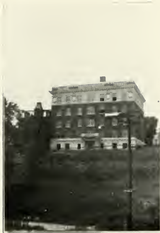
NEW BUILDING OF THE DEACONESS' HOSPITAL View from the east
