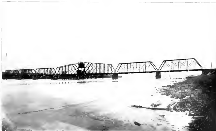
THE PEORIA & PEKIN UNION RAILROAD BRIDGE, RECENTLY SUPPLANTED BY A FIVE HUNDRED THOUSAND DOLLAR STRUCTURE
